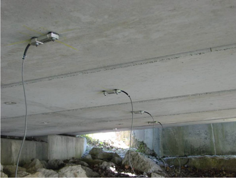
Fig. 11.12 Strain transducers attached to the underside of the bridge
