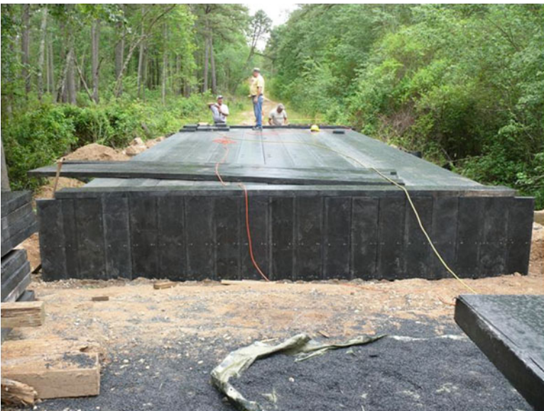
Fig. 10.23 Abutment of T85-18 finished with 3 in x 12 in boards
