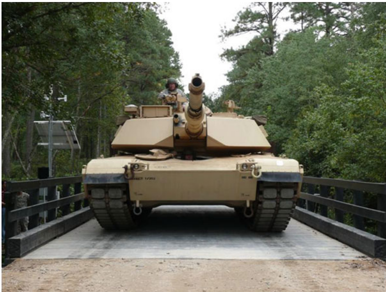
Fig. 10.24 M-1 Abrams tank (71 tons) crossing the RTCL bridge T85-18 at Fort Bragg on September 18, 2009
