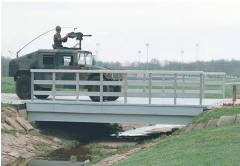
Fig. 10.3 Vehicular bridge at Fort Leonard Wood, MO built in 1998 with a maximum load capacity of 12.5 tons
