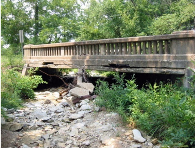
Fig. 9.4 Side view of bridge P-962
