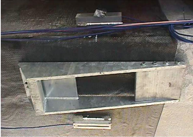
Fig. 11.11 View of anchorage system including installed sensors and FRP reinforcement
