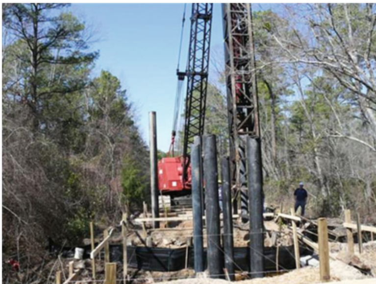
Fig. 10.16 Four-ton hammer driving piling to 37.5 ton limit
