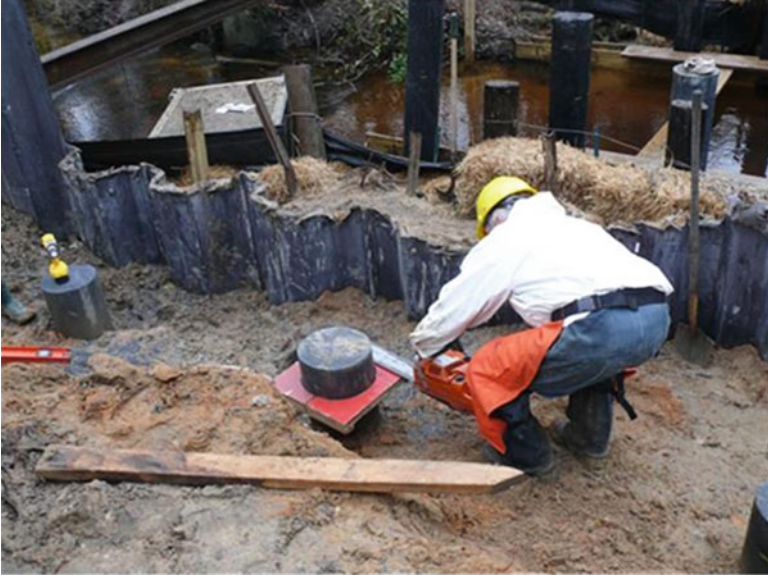
Fig. 10.18 Trimming piling to be level
