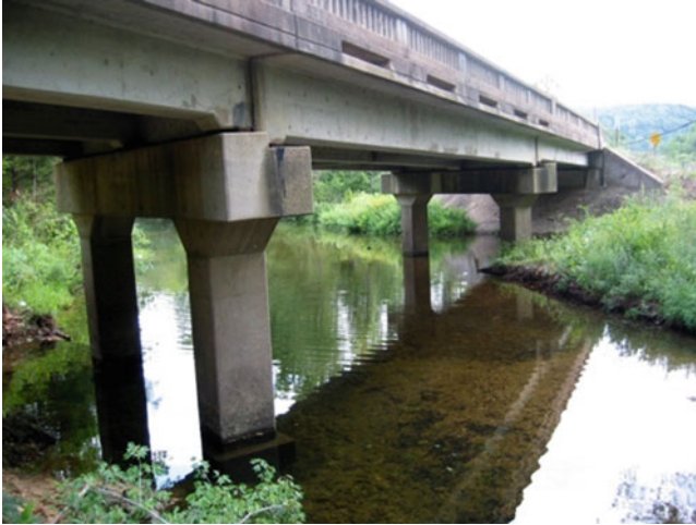
Fig. 9.3 Tested span of bridge X-495
