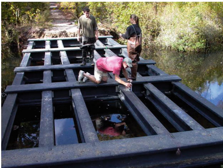
Fig. 10.5 I-beam sub-structure of the Wharton State Forest, NJ, bridge
