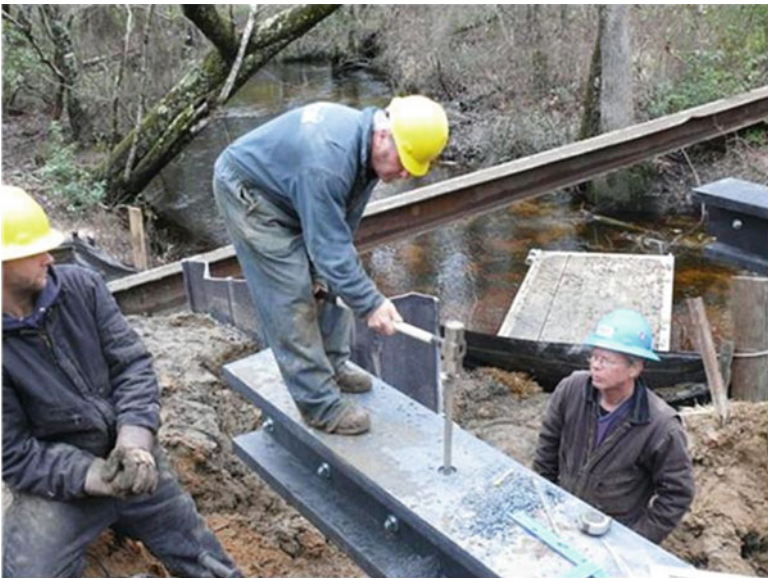
Fig. 10.19 Hammering pin through pile cap and into pile
