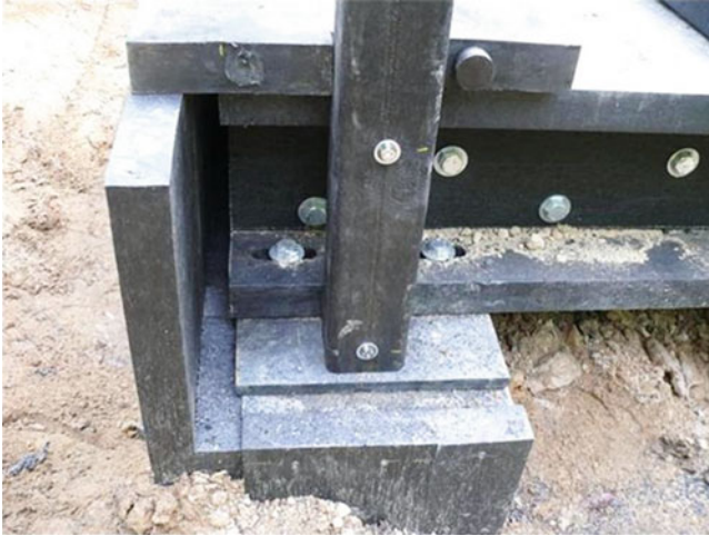
Fig. 10.13 Bridge Abutment, showing thermal expansion slots in girders
