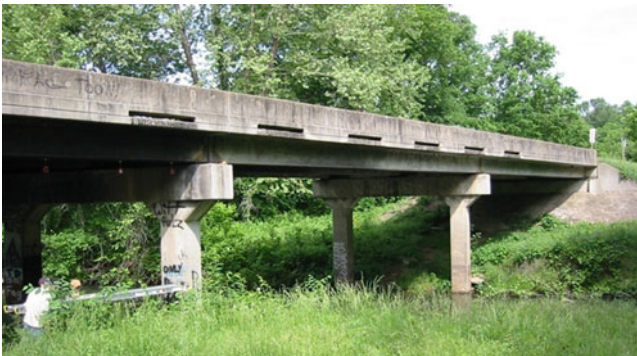
Fig. 9.5 Side view of bridge Y-298
