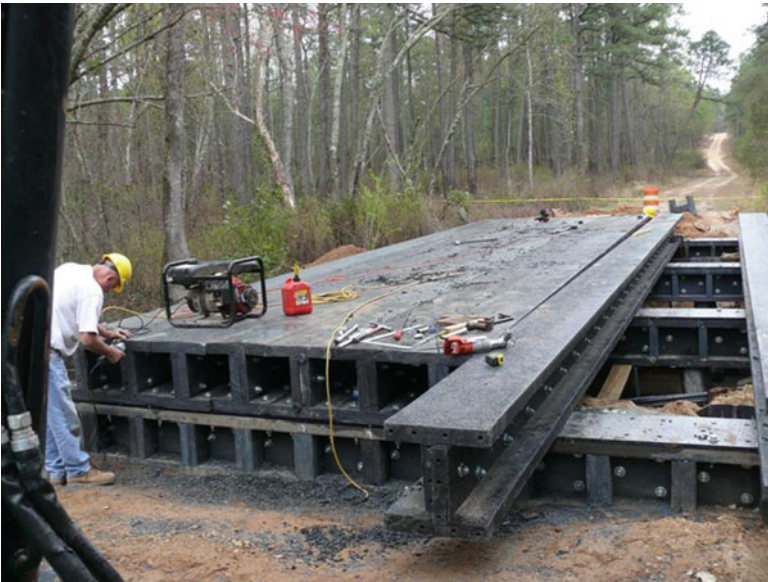
Fig. 10.9 Installation of girders on pile caps on T85-18
