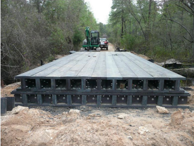
Fig. 10.10 Girders installed on T85-18 spanning the length of the bridge
