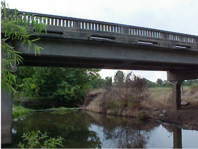
Fig. 9.1 Tested span of bridge X-596
