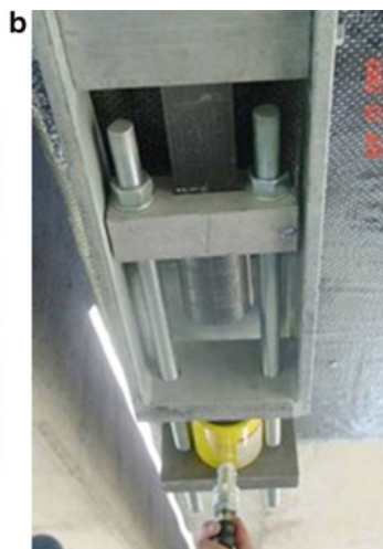
Fig. 11.2 (a) Stress head component of the CFRP strip. (b) Stressing anchor
