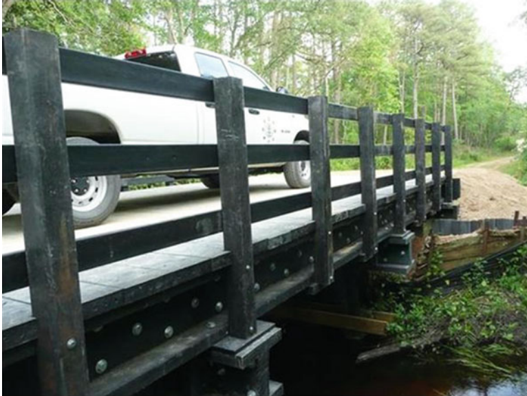
Fig. 10.12 Side of deck, showing profile of bridge with railing detail
