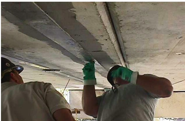
Fig. 11.10 Sika stress head S624 strip and S1012 strip (Sika 2002)
