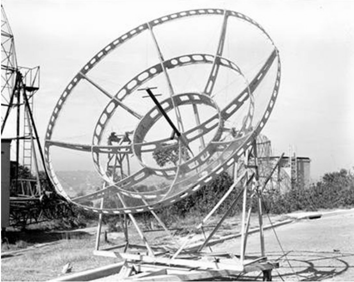
Fig. 3 A TPS-3 aerial on an improvised mount at Georges Heights field station in 1948 (courtesy: ATNF Historic Photographic Archive).
