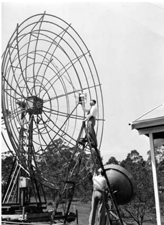
Fig. 5 The 21-ft aerial at Murraybank with its new feed system. The smaller reference aerial is also visible in the background (courtesy: ATNF Historic Photographic Archive).
