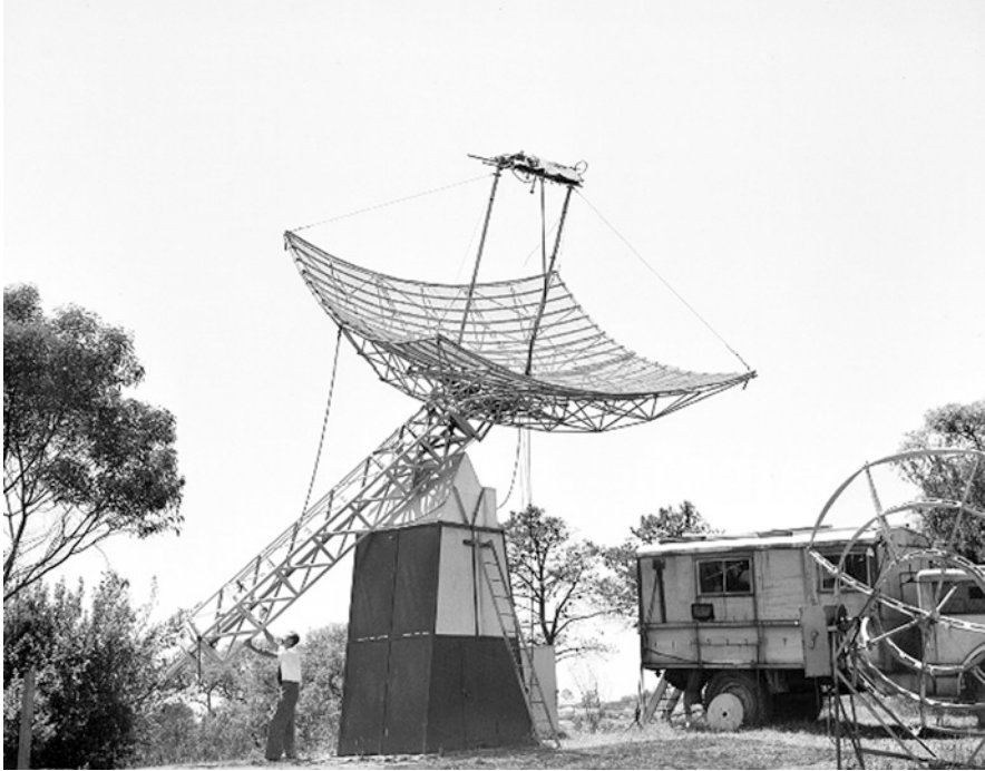
Fig. 4 The 16×18-ft antenna on its new equatorial mount at Potts Hill field station. A TPS-3 aerial is visible in the right foreground (courtesy: ATNF Historic Photographic Archive).
