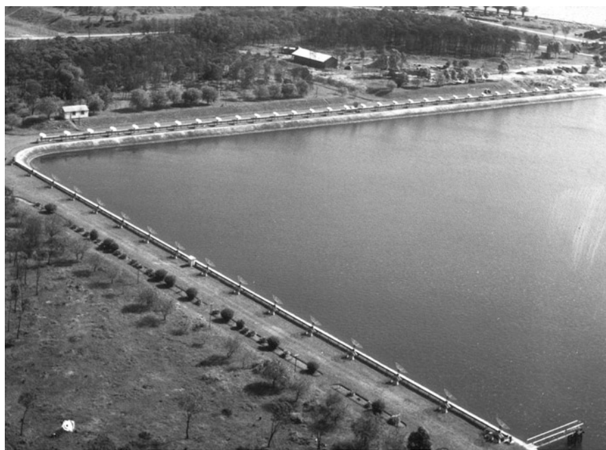
Fig. 14 Aerial photograph of the northern Potts Hill reservoir looking south-west. Along the eastern bank of the reservoir ( in the foreground ) is the 14-element grating array constructed in 1953 and along the southern bank is the original 32-element grating array constructed in 1951–1952 (courtesy: ATNF Historic Photographic Archive).
