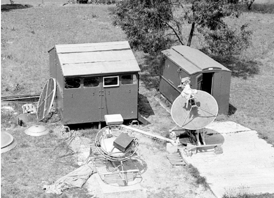
Fig. 13 The 44-in. ( left ) and 68-in. ( right ) parabolas at Potts Hill used during the 1948 eclipse and for the ongoing solar monitoring program (courtesy: ATNF Historic Photographic Archive: B3171-1R).
