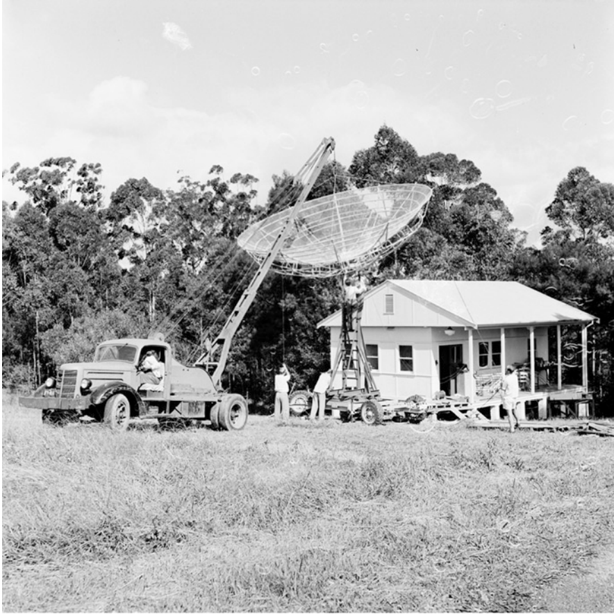
Fig. 4 The 21-ft aerial being installed at Murraybank on 18 May 1956. The equipment hut is in the immediate background (courtesy: ATNF Historic Photographic Archive B3973-4).
