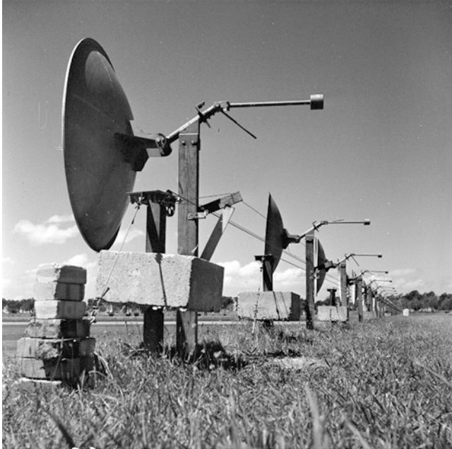
Fig. 10 The array showing the bracing weights for the open-wire transmission lines (courtesy: ATNF Historic Photographic Archive).
