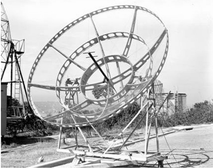
Fig. 11 An ex-WWII AN/TPS-3 aerial undergoing trials at Georges Heights on 13 August 1948 prior to being relocated to Potts Hill (courtesy: ATNF Historic Photographic Archive: B1511).
