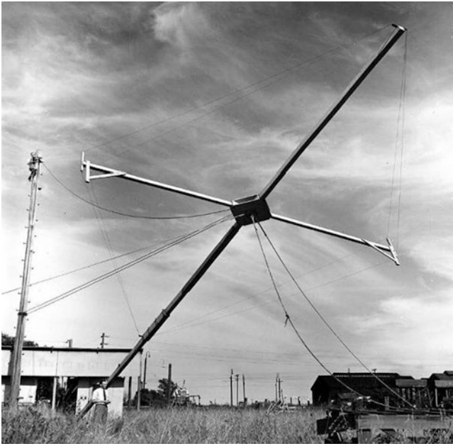
Fig. 2 The rhombic aerial and pulley system with Bill Rowe standing nearby. In the background, on the right hand side, can be seen the Penrith railway locomotive shunting sheds (courtesy: ATNF Historical Photographic Archive).
