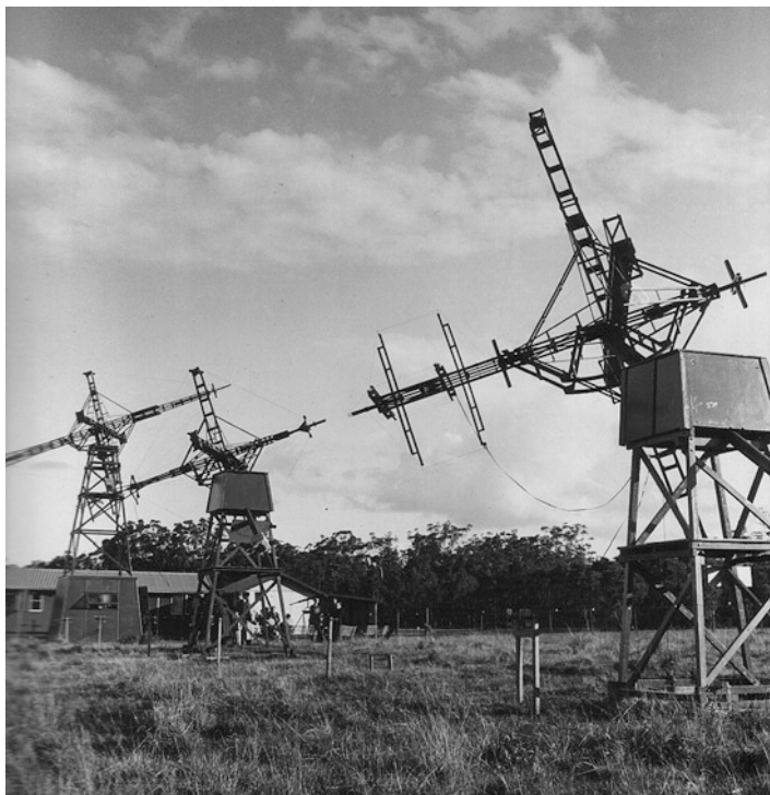
Fig. 10 The three crossed-rhombic aerials of the 40–240 MHz Radiospectrograph at the Dapto field station (courtesy: ATNF Historic Photographic Archive).
