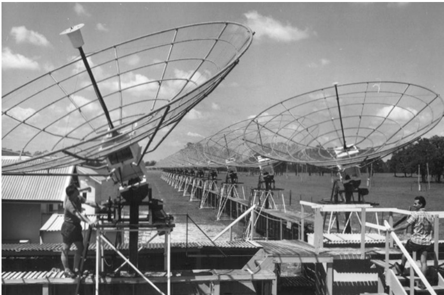
Fig. 1 The central section of the Chris Cross at Fleurs, looking south along the N-S arm. The Murraybank aerial was based on the design of one of these aerials but with an increased diameter and strengthened structure (courtesy: ATNF Historic Photographic Archive).
