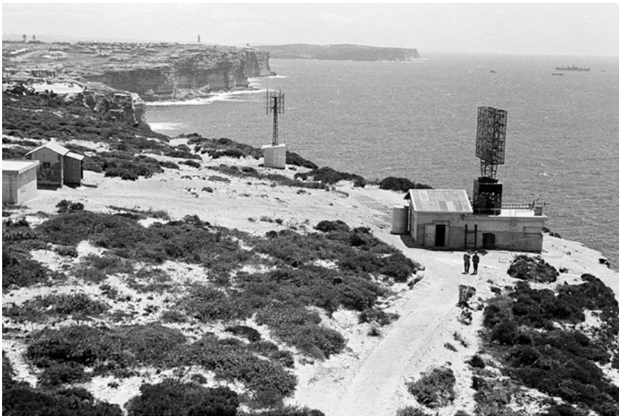
Fig. 2 The Dover Heights WWII radar station showing the seaward blockhouse containing a 200 MHz broadside array that was used at 200 MHz for solar radio observations in 1945 and 1946 (courtesy: ATNF Historic Photographic Archive).
