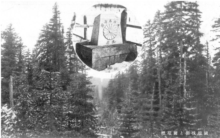
Fig. 7 The circular inset image shows one of the boundary stones, on both sides of which the national emblems of the two countries were inscribed. The main photograph shows how trees around each stone and along the border between the four stones were all removed in order to allow a clear view of the location of the border (photograph courtesy of the Otaru Museum).
