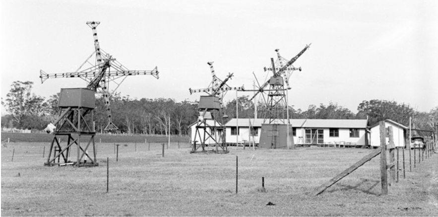
Fig. 2 Photograph of the three Dapto crossed rhombic aerals on their mounting towers, with the receiver hut in the background (courtesy: ATNF Historic Photographic Archive).
