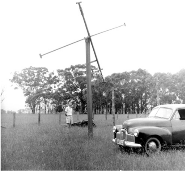
Fig. 28 Paul Wild standing near one of the interferometer rhombic antennas (courtesy: ATNF Historic Photographic Archive).
