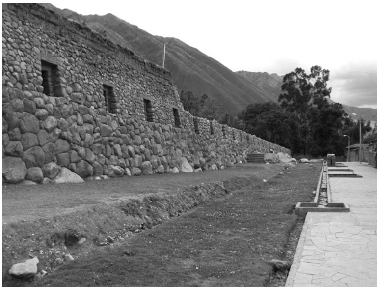
Fig. 30 Niches in Quespiwanka's south wall.
