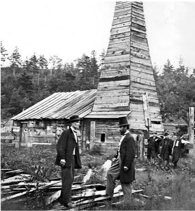
Fig. 4.1 By August 27, 1859, in the sleepy lumber town of Titusville, Pa., “Colonel” Drake hammered 10-foot sections of an iron pipe into the ground and, at a depth of 21 meters below ground, he finally struck oil. The world changed forever. Over a century and a half, Drake’s 25 barrels-per-day well would give rise to the world’s largest industry. Globally, the industry now produces 73 million barrels per day, making oil the world’s most strategic commodity, supplying 40% of the world’s energy. (Source: eworld.com/article.cfm?storyid=1749 )
