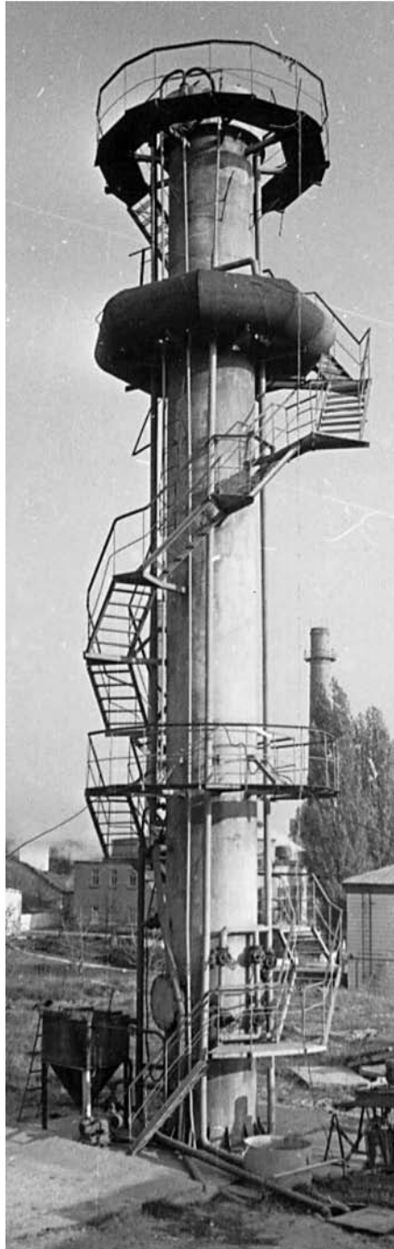
Fig. 9.7. View of the pilot plant combining columnar aeration tank-clarifier with tertiary filtration in a single reactor.
