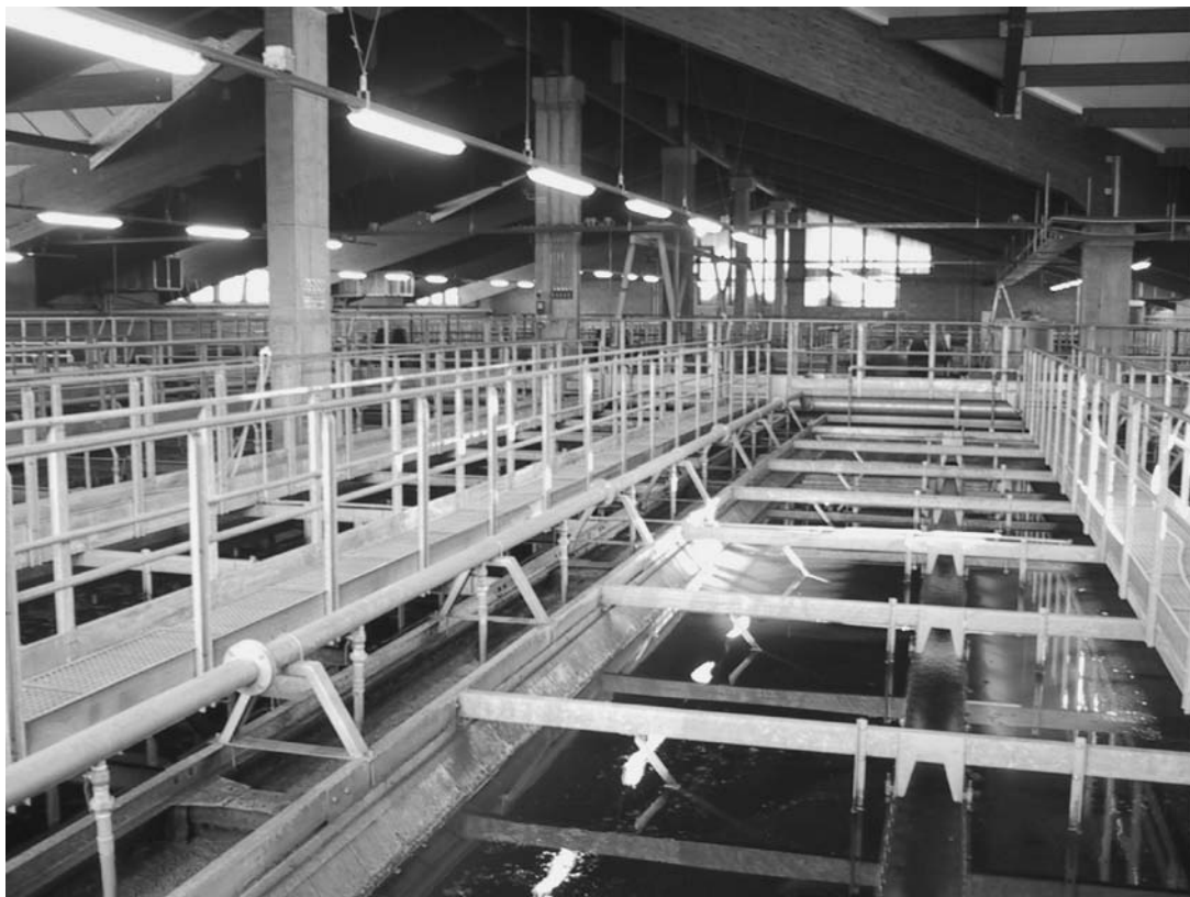
Fig. 10.26. Picture of USBF reactor in WWTP Pinzolo (Italy) after upgrading to COMBI USBF.
