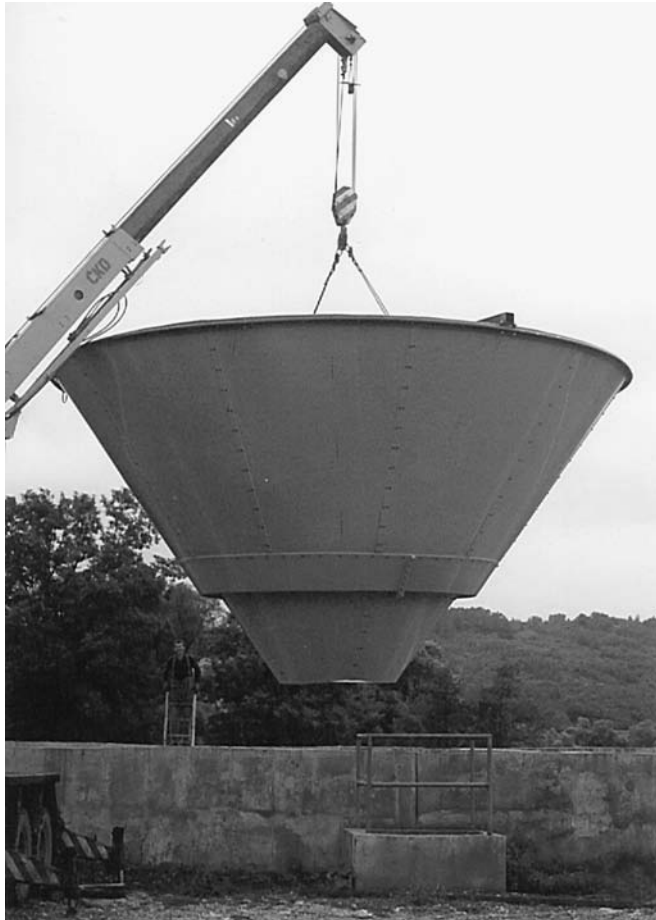
Fig. 10.23. Picture of the funnel-shaped COMBI USBF separator.
