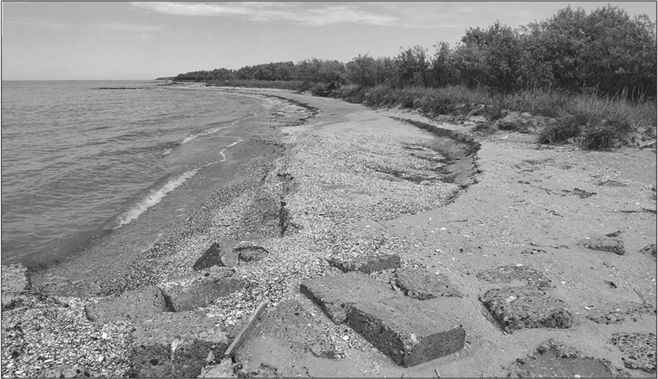
**Fig. 5.38** The dike dam protects the beach from erosion on the western shore of the Chushka spit (Photo by V. Krylenko)
