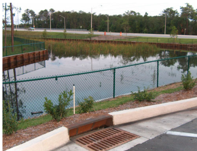
Fig. 11.12 An artificial wetland to treat runoff from a commercial parking lot in Florida. The plantings primarily consist of cattails and sedges, as seen in the middle of the water, with willows along the banks (Photograph by author).
