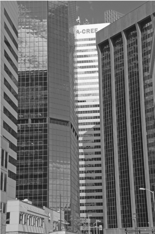
Figure 3.18. As curtain wall technology evolved, the use of operable windows gave way to HVAC control. The only fresh air came in through the mechanical system.
