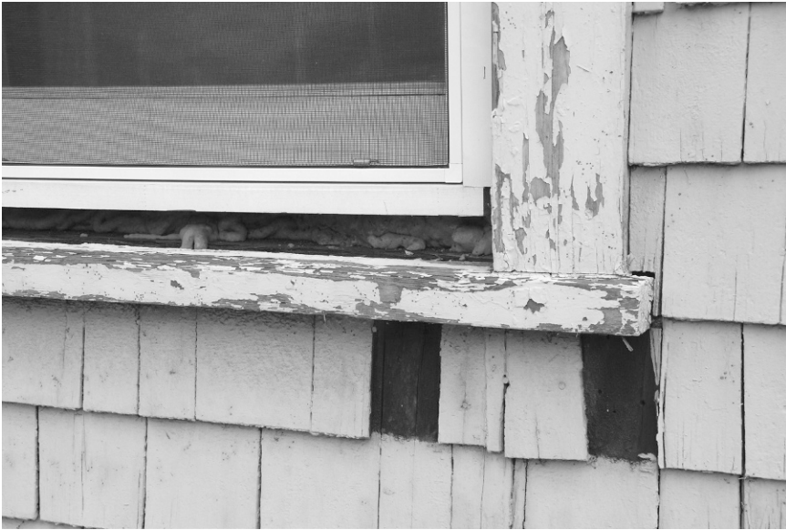
Figure 3.26. Foam insulation products will seep through any gaps that they can. There are insulation foam products with expansion rates specifically formulated for use in finished cavity walls.
