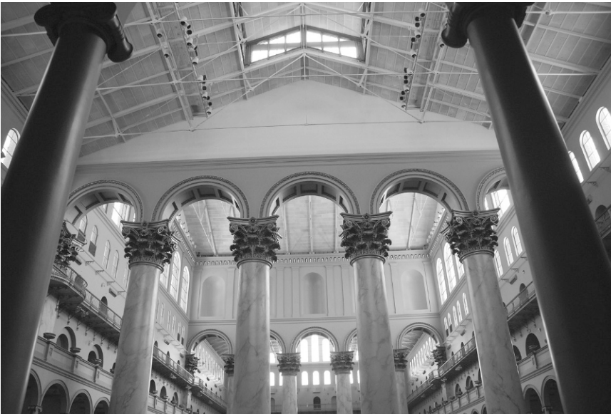
Figure 3.14. The Pension Building, completed in 1887 in Washington, DC, shows how the stack effect and cross-ventilation were integrated into commercial buildings. (Photo: © R. A. Young, shown here with permission of the National Building Museum.)
