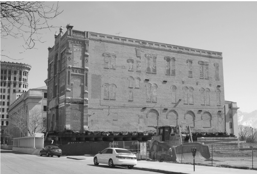
Figure 3.2. The Odd Fellows Hall in Salt Lake City, Utah was saved from demolition by moving it across the street.
