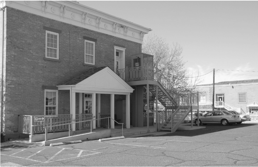
Figure 1.9. The Americans with Disabilities Act mandates accessibility upgrades to public buildings. One solution has been to redefine the main entrance as adjoining the parking lot (commonly at the rear of the building), where access for the disabled can be achieved more readily without compromising the historic features of the traditional front entrance. Shown here is the Washington County Courthouse in St. George, Utah.
