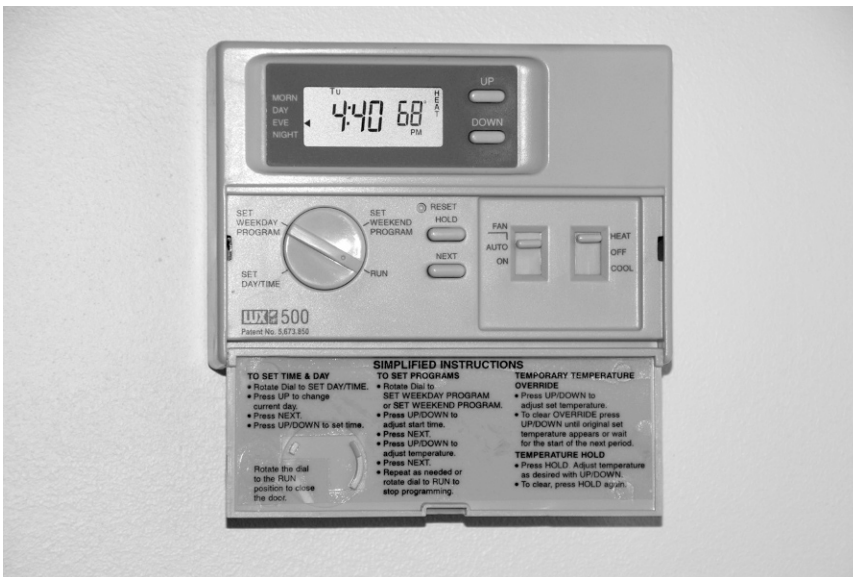
Figure 3.30. Programmable thermostats have been proven to be an effective means to reduce energy use and costs. Payback periods of less than 1 year are common.
