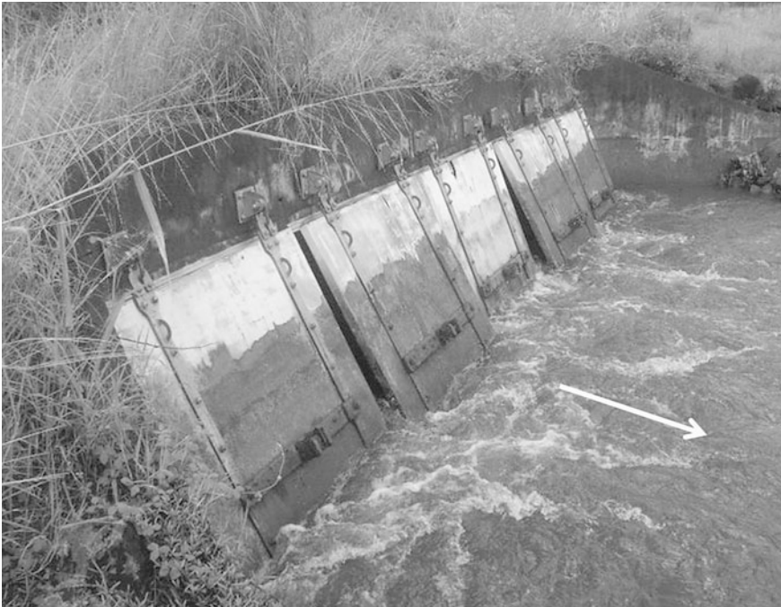
FIGURE 17.1. Typical top-hinged tidal floodgates. Ebb tide flow is indicated by the white arrow. The floodgate flap remains closed when downstream water levels are higher (due to tides or flooding) than upstream water levels. When upstream water levels are higher (due to low tides, large inflows, or backswamp flooding), hydrostatic pressure forces the floodgate flap to open.
