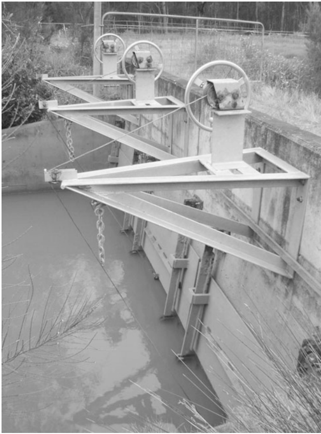
FIGURE 17.2. Example of modified cantilever floodgates.
