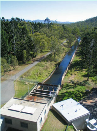
Box Fig. 3.3b.1 Irrigation scheme in South-East Queensland (Photo credit: Veronica Strang)
