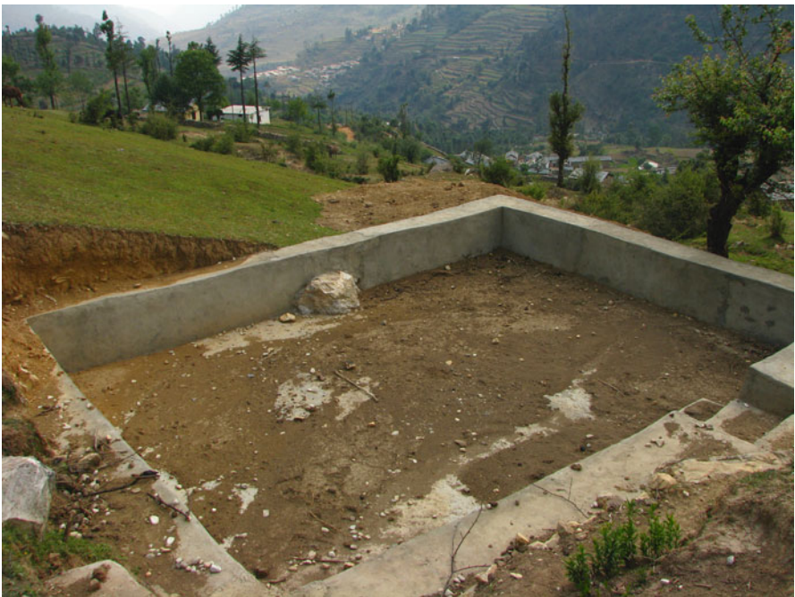
Fig. 5.1.2 A chaal in Thaandi village, Dunda block, Uttarakashi, constructed with NREGA funds (Photo credit: A. Acharya)
