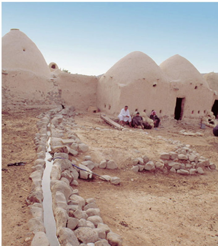
Fig. 2.3.2 Open channel in qanat community in North West Syria (Photo credit: Joshka Wessels)
