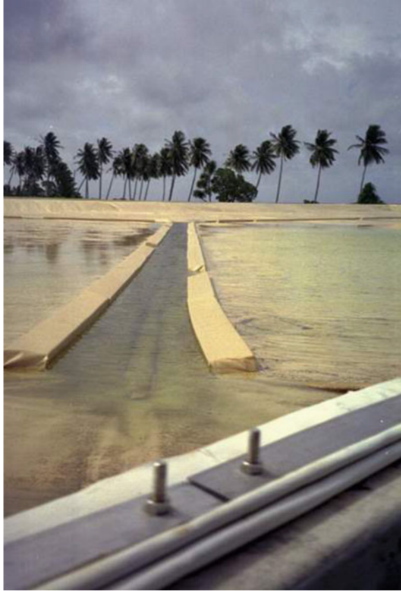
Fig. 3.4.1 Freshwater reservoir created by runoff from Majuro airport, Marshall Islands (Photo credit: Barbara Rose Johnston)
