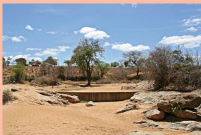
Box Fig. 2.2a.2 A sand dam during the dry season (Source: NWP 2007)
