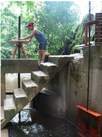
Fig. 1.4.6 Opening the irrigation gate, Ecuador, Chimborazo province (Photo credit: Rutgerd Boelens)
