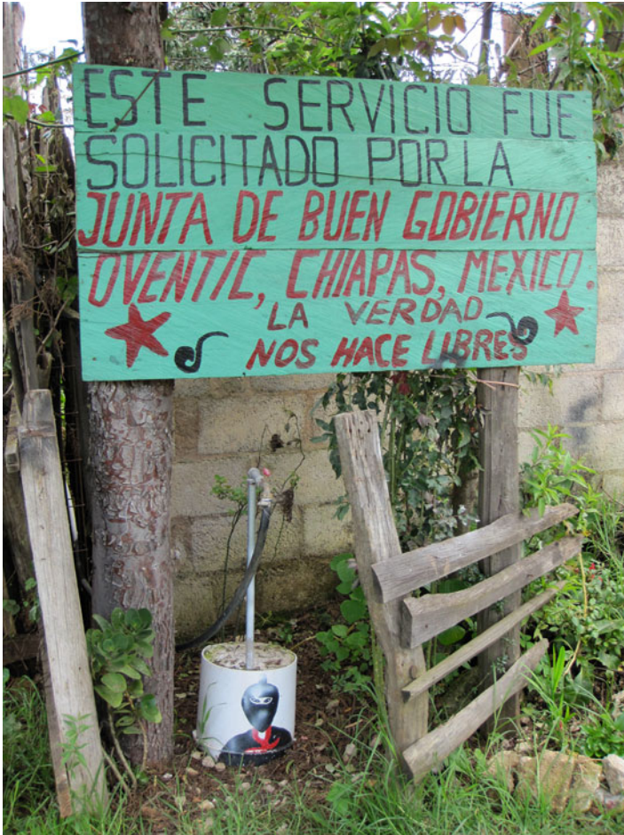
Fig. 2.5.1 A Zapatista public hydrant in Cinco de Marzo. Translation of sign: This service was commissioned by Council of Good Government in Oventil, Chiapas, Mexico. The truth sets us free. (Photo credit: Ameyali Ramos Castillo)
