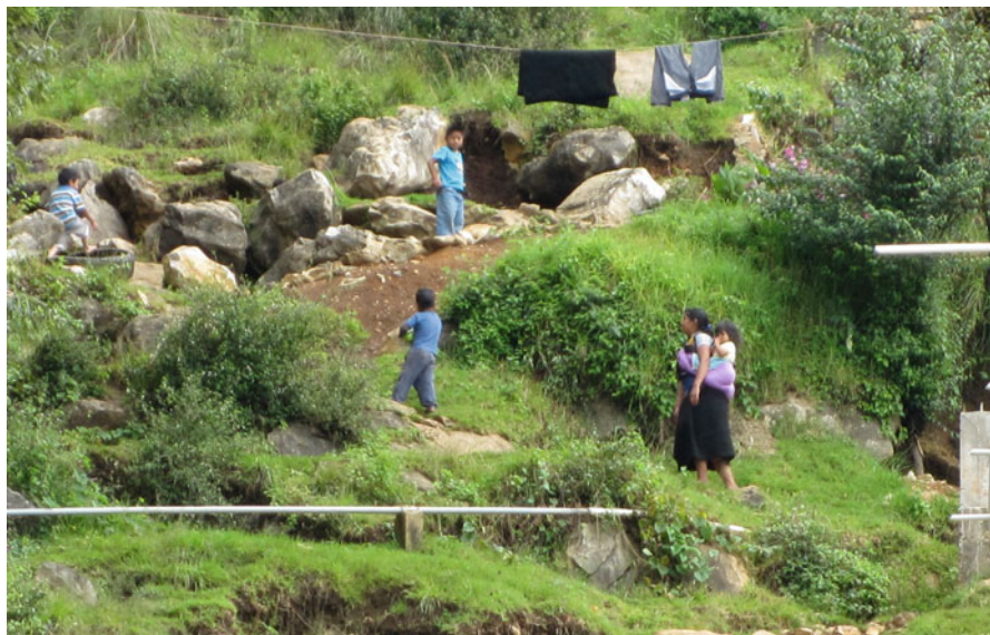
Fig. 2.5.4 Pipes carrying water from El Pinar to La Hormiga (Photo credit: Ameyali Ramos Castillo)
