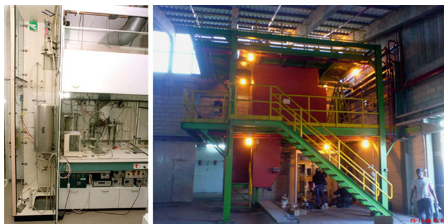
Fig. 27.4 Production facility for 20 g/batch ( left ) of IF-WS 2 erected in 2000 and a pilot for 150 kg/batch of industrial grade IF-WS 2 nanoparticles ( right ) in “NanoMaterials” site
