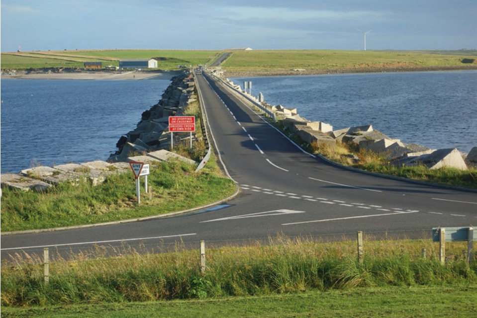
Fig. 7.6 This photograph from August 2015 shows Churchill Barrier Number One, which now completely blocks the Kirk Sound channel through which the U-47 entered Scapa Flow (Photograph by the author)
