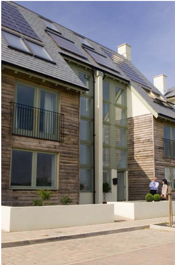
Fig. 10.2 Solar panels on houses at Upton. Photovoltaic panels (electricity producing) and Solar thermal panels (hot water producing) on houses at Upton
