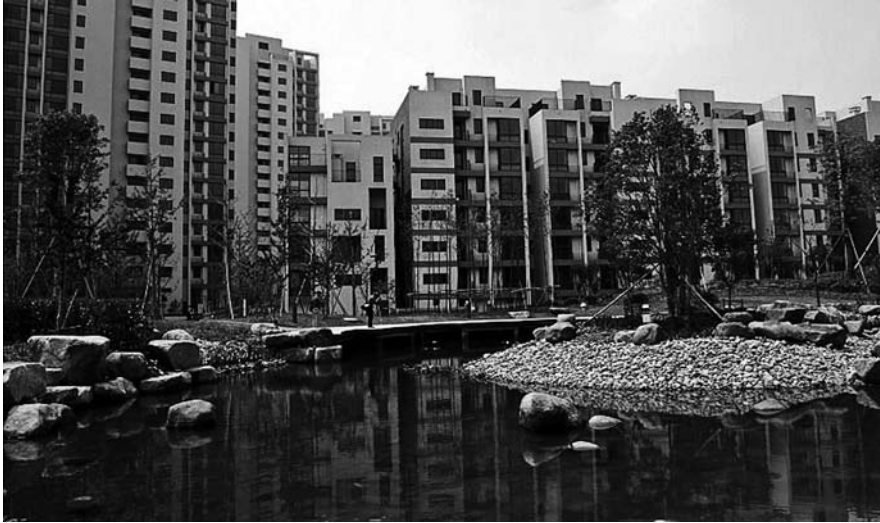
Fig. 15.3 Skyscrapers. An example of an ecologically designed residential compound. From now on, almost all Jiaxin's newly built residential areas are designed and planned with ecological and energy-saving considerations
