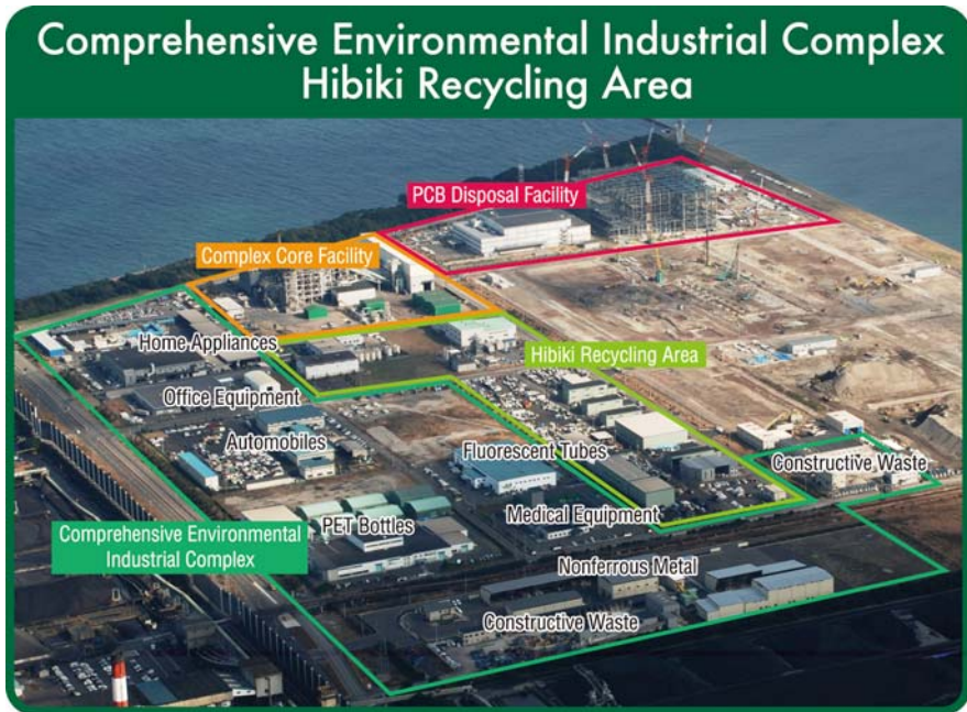
Fig. 16.1 Comprehensive Environmental Industrial Complex, Hibiki Recycling Area, Kitakyushu City, Fukuoka, Japan
