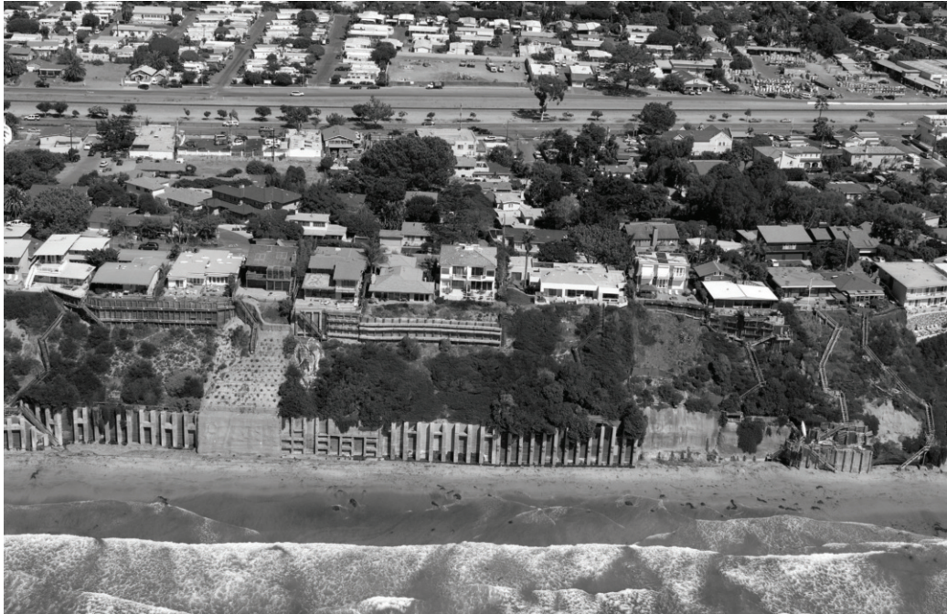
Figure 9.8 Coastal armoring in Southern California. One-third of the shoreline of Southern California (including Ventura, Los Angeles, Orange and San Diego Counties) has now been armored. The photo shows the shoreline in 2010 in Encinitas, in northern San Diego County. Photo courtesy of Kenneth and Gabrielle Adelman of the California Coastal Records Project ( http://www.californiacoastline.org/ ).
