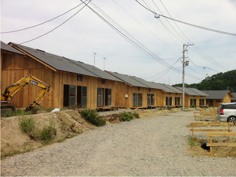
Fig. 4.6 Wooden temporary housing constructed using local materials in Iwaki city
