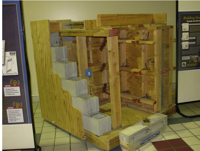
FIGURE 2-5 Tulsa, Oklahoma, November 23, 2001. Disaster Ally in the Eastland Mall. Safe rooms can be designed with many different materials. Shown are concrete block walls, formed concrete walls, and a special ceiling framing. Photo by Kent Baxter/IFEMA News Photo.
