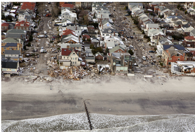
FIGURE 2-1 Long Beach, N.Y., Nov. 8, 2012—Aerial views of Hurricane Sandy damage to homes on Long Beach, New York. Following the hurricane, a nor'easter struck the area causing more power outages and additional flooding. FEMA is working with state and local officials to assist residents who were affected by Hurricane Sandy. Andrea Booher/FEMA.
