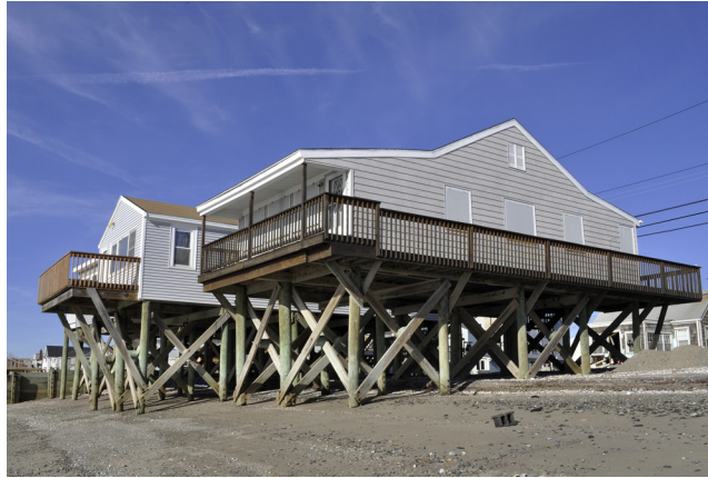
FIGURE 3-1 Stratford, Connecticut., December 6, 2012—These summer cottages are examples of homes not severely damaged by Hurricane Sandy due in large part to being elevated on pilings. FEMA is in the area with mitigation specialists who are knowledgeable about the value of pilings to support coastal homes. Photo by Marilee Caliendo/FEMA.
