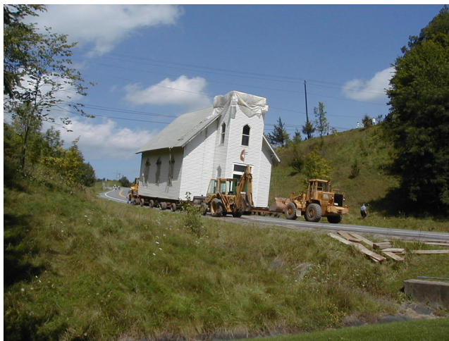
FIGURE 3-5 Albany, New York. This church is being moved half a mile to higher ground as part of the Stryker Road relocation project in Schoharie County, New York. The Hazard Mitigation Grant and Public Assistance Programs helped fund the project. Schoharie County Planning and Development Agency photos.
