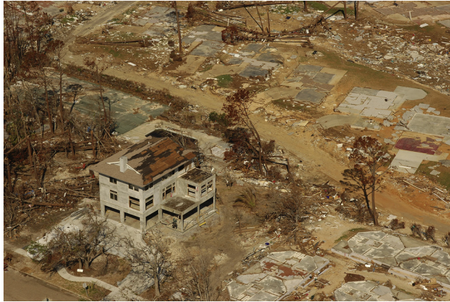
FIGURE 3-2 Pass Christian, Mississippi, October 4, 2005. Aerial photo of the only surviving home in the area that was completely destroyed by Hurricane Katrina. Foundations are all that remain of most of the neighboring homes. The surviving home was built using many FEMA standards. John Fleck/FEMA.
