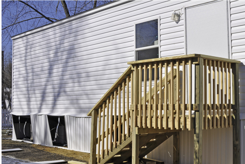
FIGURE 7-4 Freehold, New Jersey, January 27, 2013—In Freehold, New Jersey, new front steps and an entry have been attached to a Temporary Housing Unit (THU) provided by FEMA for use by a family displaced by Hurricane Sandy. THUs are administered through FEMA's direct housing program. Photo by Sharon Karr/FEMA.
