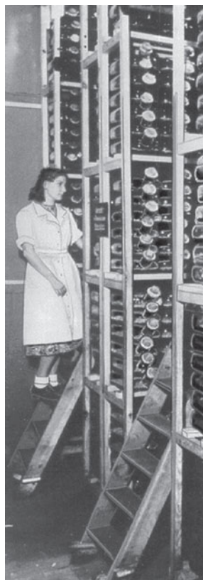
5.25 After the Second World War, penicillin was prepared batch-wise in flat glass bottles, which were stacked up in large racks.
