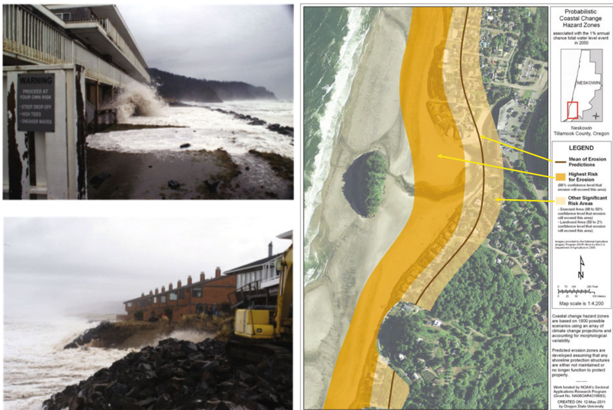
Figure 4.10 Recent coastal flooding (Allan et al. 2009), erosion, and failures of coastal protection structures in the community of Neskowin, Oregon. Both photographs were taken by Jonathan Allan of the Oregon Department of Geology and Mineral Industries (DOGAMI) in 2008 at approximately the location of the red star (right hand panel), within a shaded “coastal change hazard zone” (Ruggiero et al. 2011; Baron et al. 2010). These zones have been incorporated into Tillamook County, Oregon’s Coastal Change Adaptation Plan (Rhose 2011). Hazard zones were developed for both the annual and 100-year storm events for the time periods of 2009, 2030, 2050, and 2100. Coastal change hazard zones were derived from 1,800 scenarios using an array of climate change projections and accounting for coastal morphological variability.
