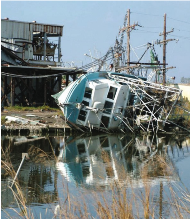
Figure 9.1 A fishing vessel lies on its side near a wholesale fishing dock in St. Bernard Parish, Louisiana, after Hurricane Katrina. Adjacent infrastructure also suffered massive damage. Photo by Paula Ouder. Courtesy of Louisiana Sea Grant College Program.
