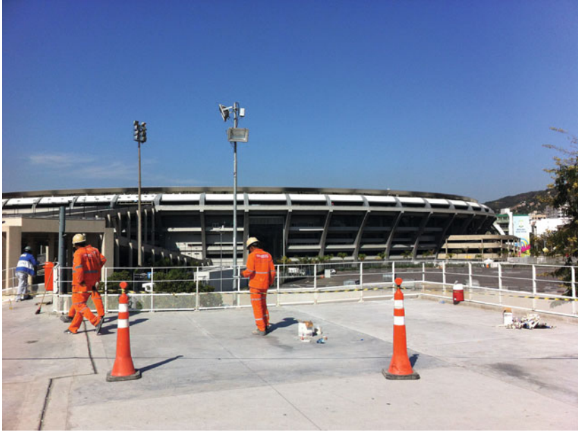
Fig. 11 The Maracanã stadium, under renovation
