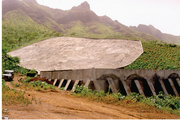
Fig. 6.3 Rainwater harvesting for village domestic water supply in Cape Verde (courtesy by Angela Moreno)
