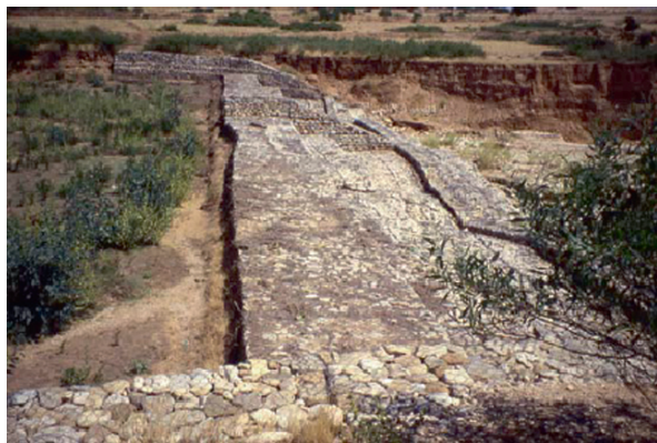
Fig. 7.7 Gabions recharge dam in a wadi, Central Tunisia
