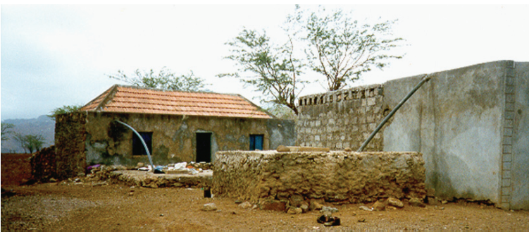
Fig. 8.7 Roof-top rainwater harvesting in Cape Verde (courtesy by Angela Moreno)
