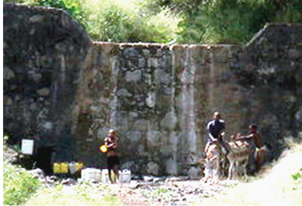
Fig. 5.2 Capturing water from a check dam in a torrent gully
