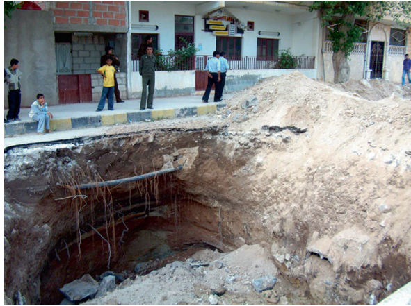
Fig. 7.3 Sinkhole formed due to drawdown of the aquifer at Ras-El-Ain, Syria (courtesy by Nicola Lamaddalena)
