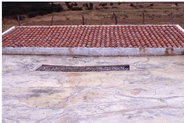
Fig. 6.4 Rainwater collection area with a filter as used in Northwest Brazil
