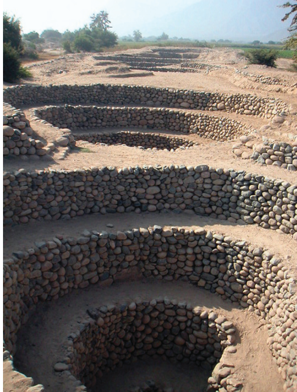
Fig. 5.5 The Nasca aqueducts for capturing groundwaters flowing from the Andes to the arid coastal area in southern Peru
