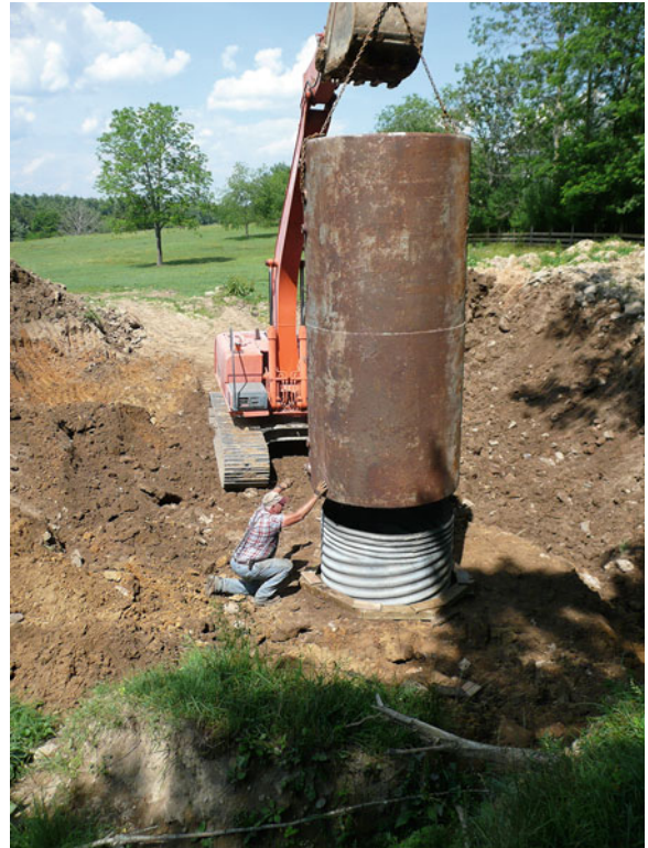
Fig. 13.13 Installing the tank. Photo by P. C. Lucas
