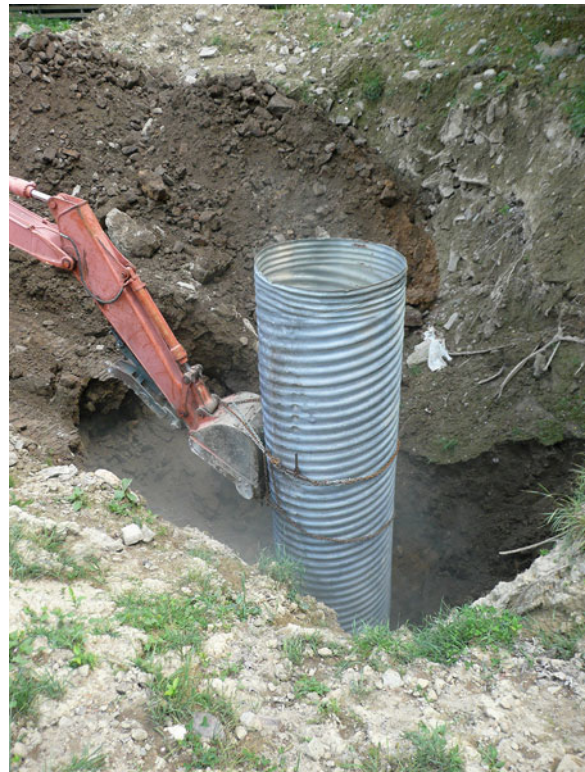
Fig. 13.11 Installing the culvert. Photo by P. C. Lucas
