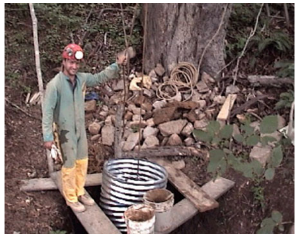
Fig. 9.16 Installing the culvert in Basswood Cave. Photo by Philip C. Lucas
