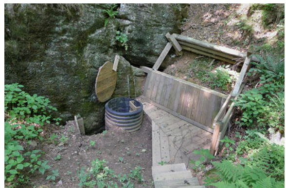
Fig. 11.49 The completed Talus Cone Entrance (photo by P. C. Lucas)
