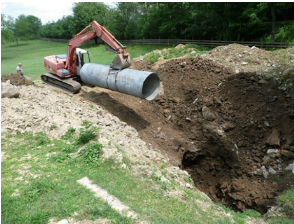
Fig. 13.10 Lifting the culvert. Photo by P. C. Lucas
