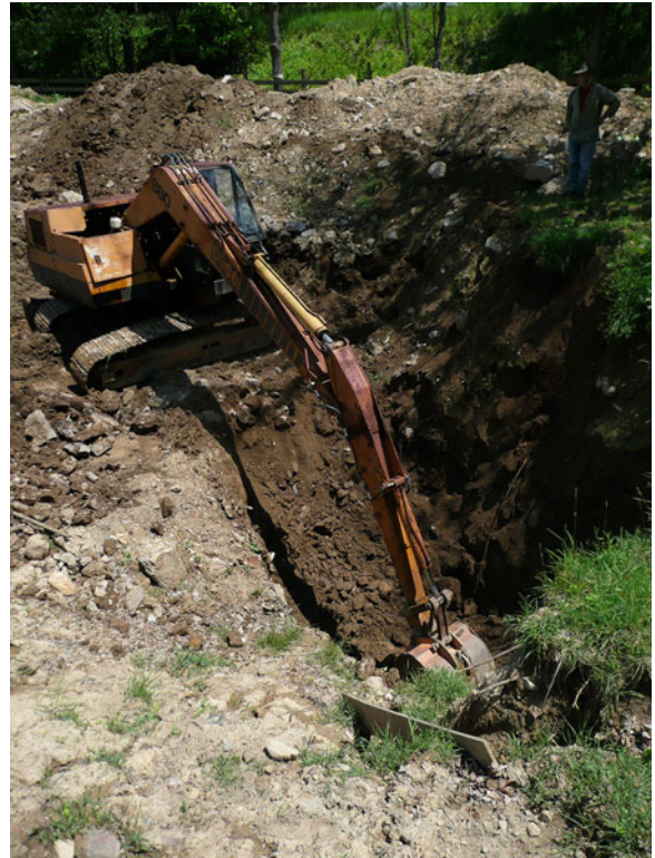
Fig. 13.8 The trackhoe reaches its limit. Photo by P. C. Lucas
