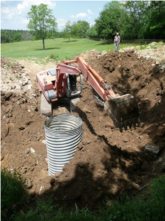
Fig. 13.12 Backfilling the culvert. Photo by P. C. Lucas
