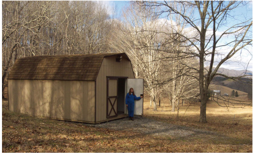
Fig. 10.9 The building over the entrance to Big Bucks Pit, December, 2012
