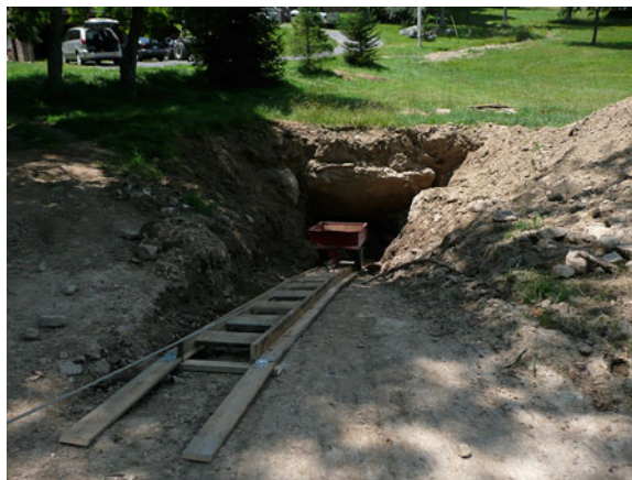
Fig. 13.5 The haul system. Photo by P. C. Lucas
