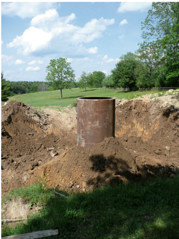
Fig. 13.14 Backfilling the tank. Photo by P. C. Lucas
