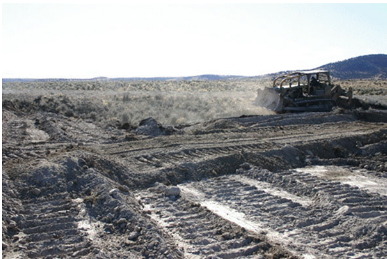
Fig. 15.2 Restoration of disturbed seasonal pool by regrading and infilling dugout
