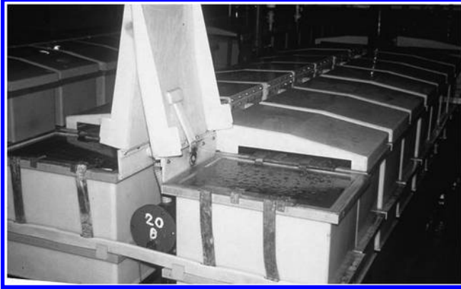
FIGURE 7.20 Lead-acid battery formation tank. (From http://www.flickr.com/photos/flexpro/sets/72157616389278240/detail/ )
