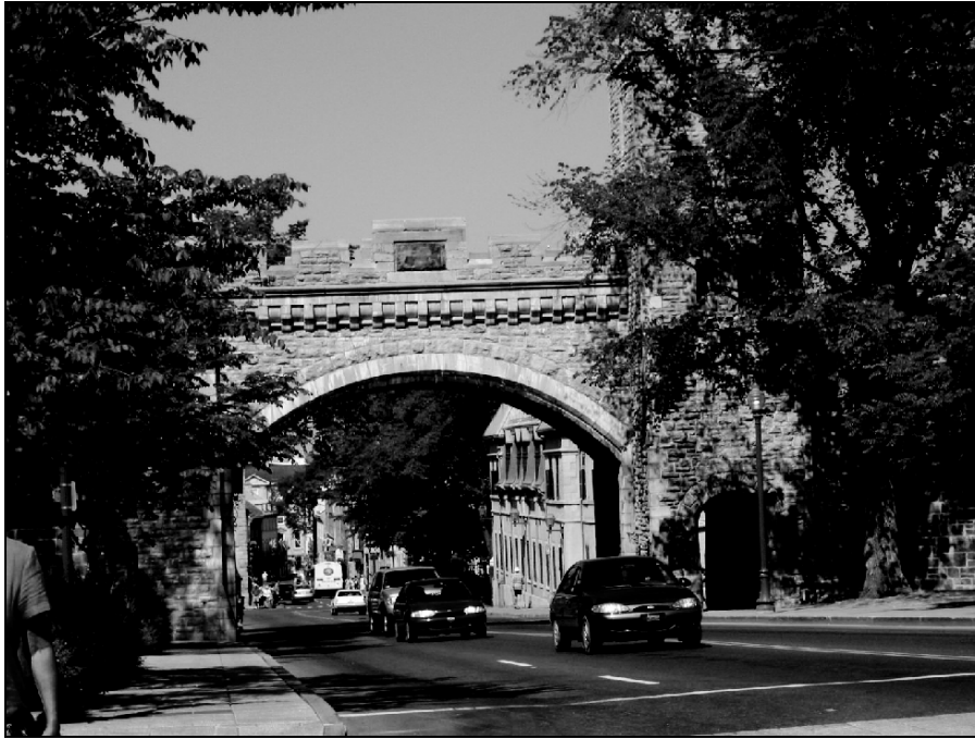
Figure 7. Porte Saint-Louis, Upper Town, M. Delisle 2003
