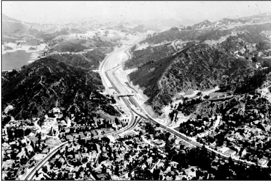
Figure 3. Construction of the Hollywood Freeway, Los Angeles, California (Spence Photo Archives, UCLA).
