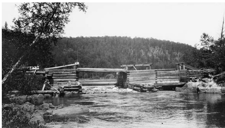
Figure 12. Dam in Algonquin Park, Ontario used for driving logs in spring.
