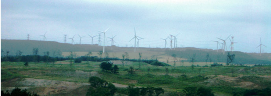
Fig. 9.3 Wind power stations in Shimokita Peninsula, Aomori, Japan
