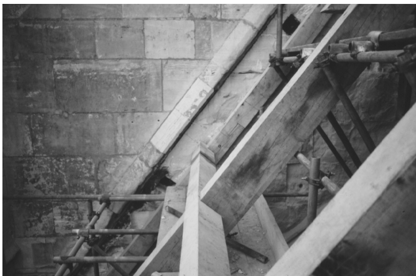
Fig. 18.7.13 The dripstone on the central tower generates the basic roof line. Small variations along the length can be sweetened by varying the depth of the truss notches to receive the purlins
