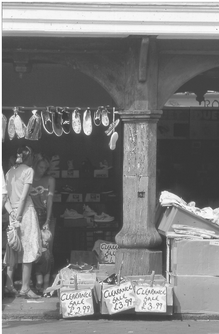
The Guildhall, Faversham. The arcades of the Guildhall date from 1574. A simple half-lap nineteenth century repair can be seen to the base of the post.
