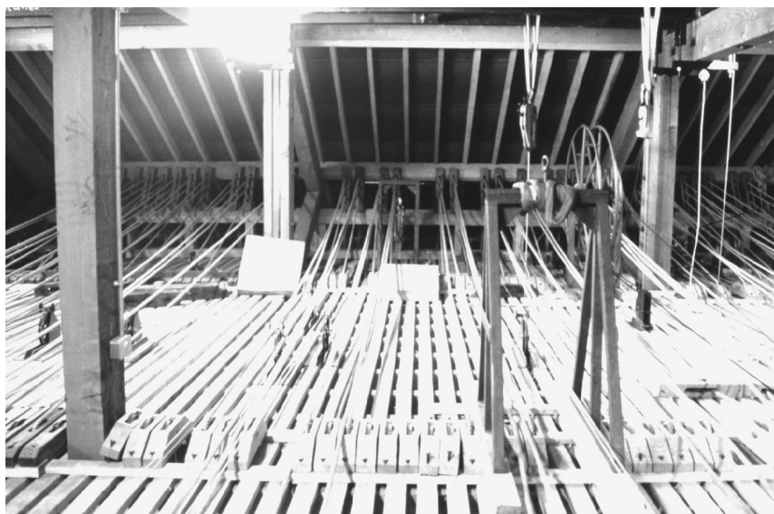
Fig. 18.6.11 Roof complete with sarking felt above and the fly tower grid rebuilt on the bottom members of the trusses
