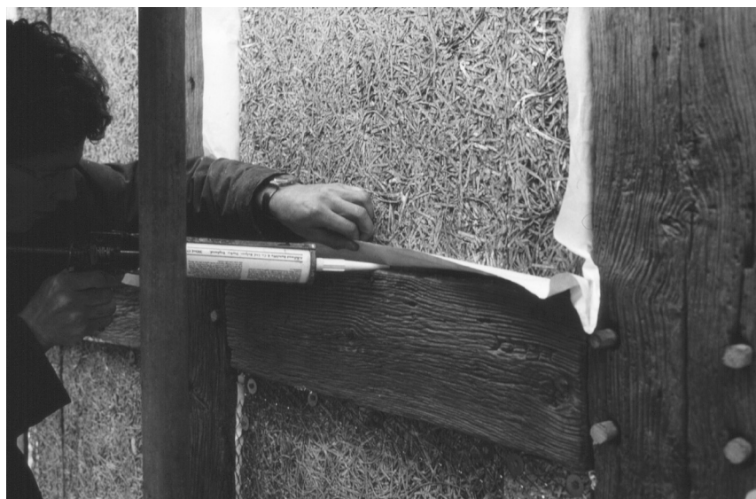
Fig. 18.5.10 Panel sealant
