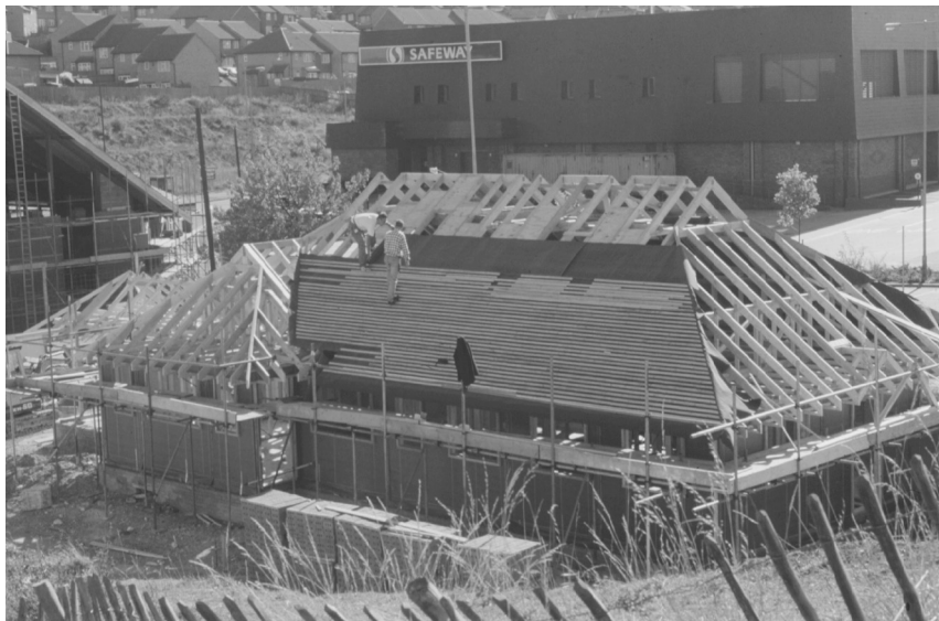
Fig. 2.12 Trussed rafters. Church, Walderslade, Kent
