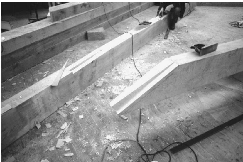
Fig. 18.6.8 Truss assembly. The joint between a principal rafter (to the left) and the mid-height collar (to the right)
