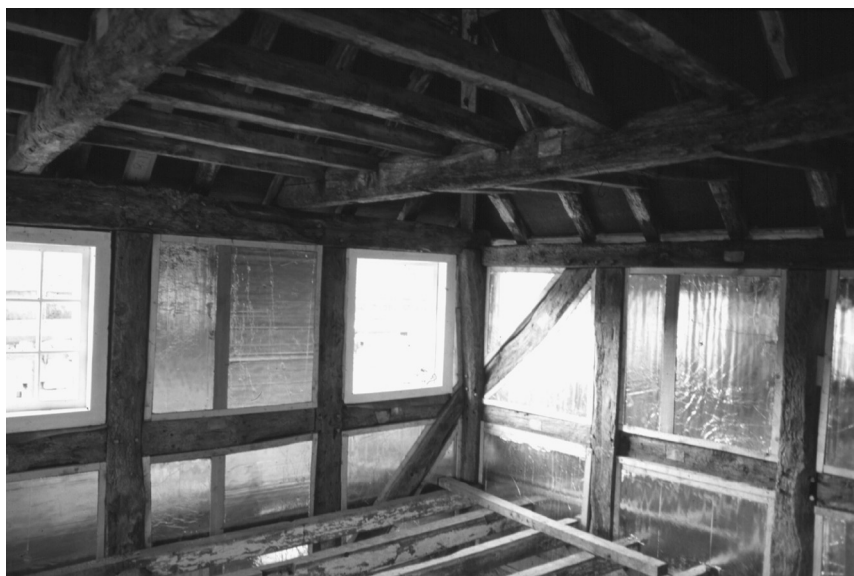
Fig. 18.5.11 Internal view of the frame, infilled with foil-backed plasterboard
