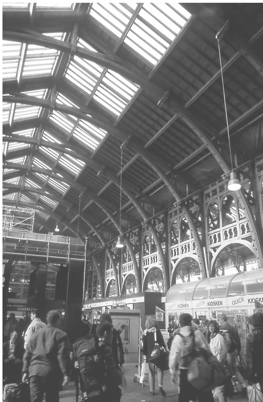
Concourse roof, Main Railway Station, Copenhagen, Denmark. Europe's best bolted laminated roof; one hundred foot span arches dating from 1901.
