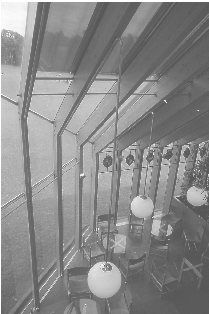
Burrell Museum, Glasgow. Softwood glulam frames, glazed externally and neatly turning the corner of the restaurant.
