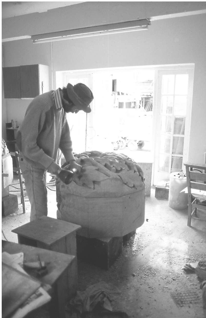
York Minster, South Transept Roof boss. Carving one of the vault bosses from a block of glued laminated oak.
