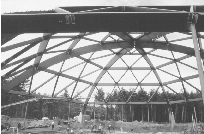
Fig. 2.13 Dome, 70 m span, of glued laminated timber, at Center Parcs, Sherwood Forest
