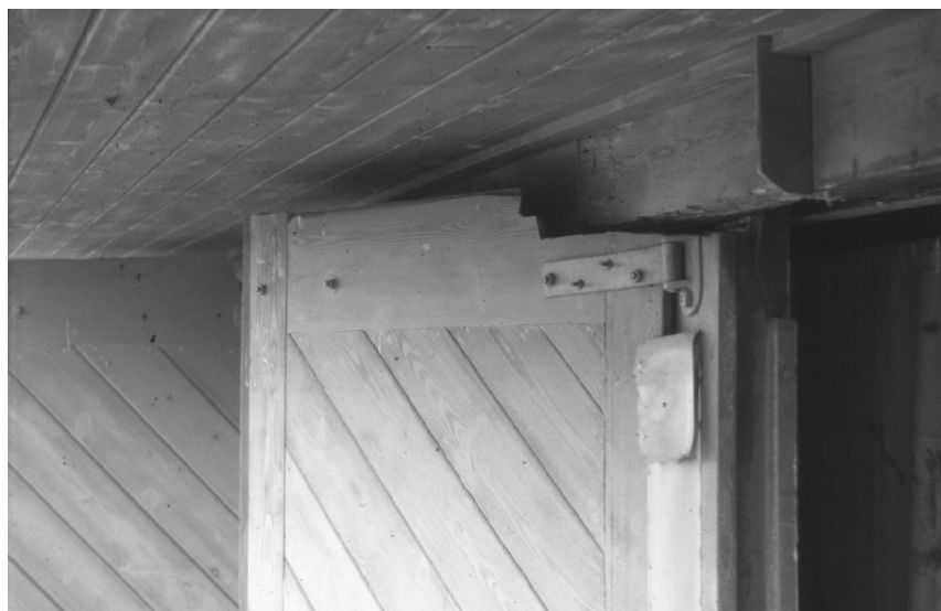
Fig. 18.1.6 Door head notched by 80 mm to accommodate the deflecting guide rails
