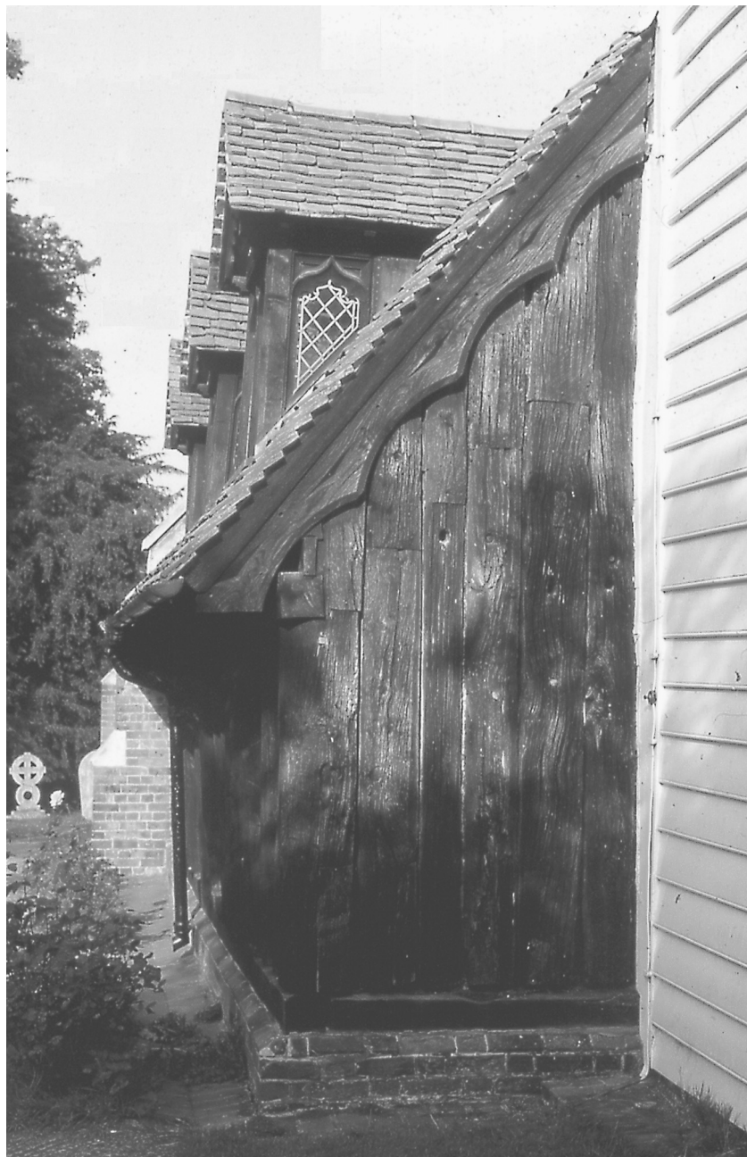
The Church of St. Andrew, Greensted-juxta-Ongar, Essex. Perhaps the oldest standing timber building in the UK, dating from around 1000 AD, and the only surviving example of vertical oak staves.
