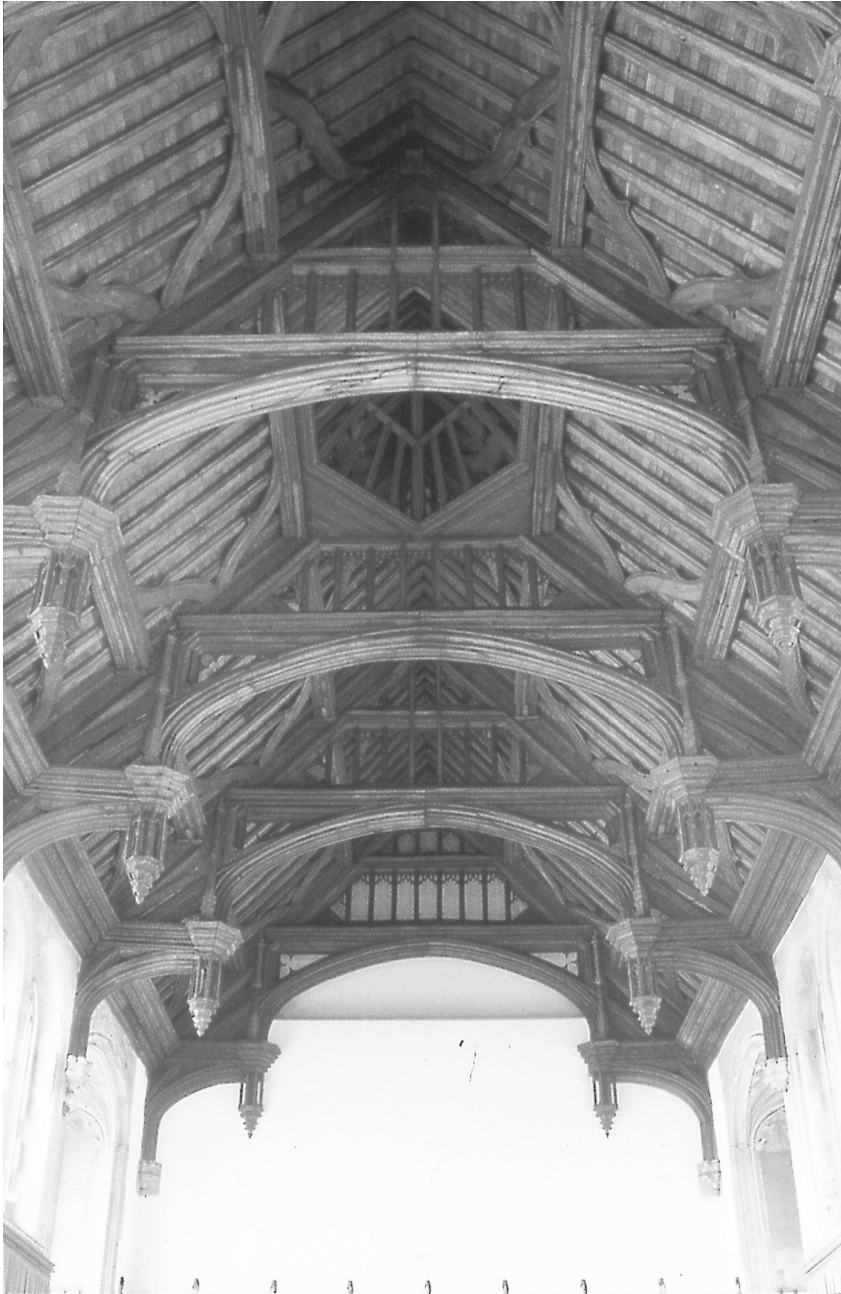
Eltham Palace, London. The hammer-beam roof of the Great Hall, begun by Edward IV in 1475.
