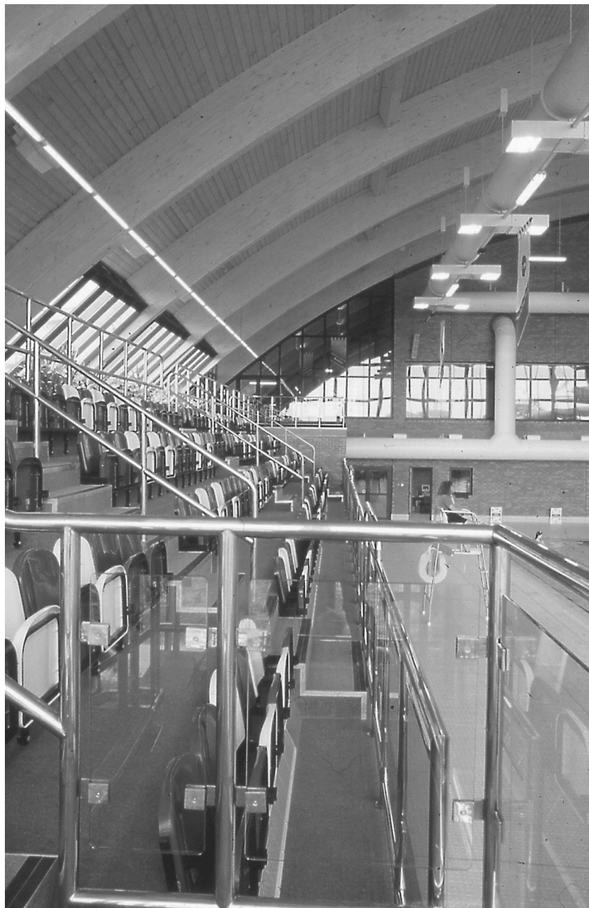
Littledown Sports Centre, Bournemouth. A forty metre span roof of three-pin glued laminated arches, with a boarded roof of solid timber, built in 1984.
