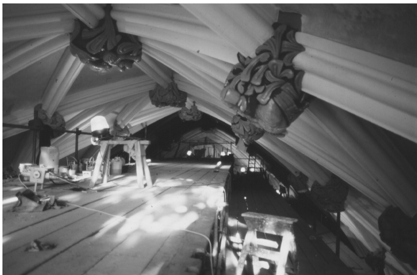
Fig. 18.7.14 Finishing work to the crown of the vault
