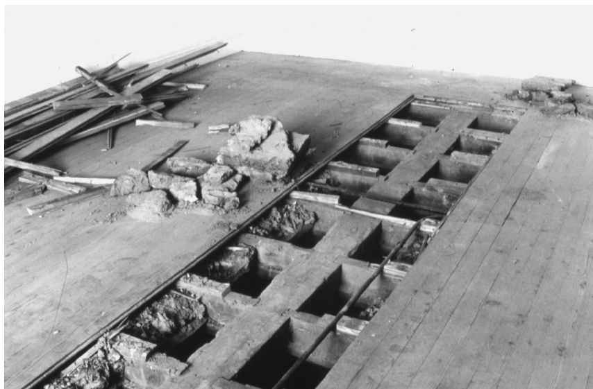
Fig. 18.2.3 Floorboards removed locally, exposing a principal beam with the common joists dovetailed into it
