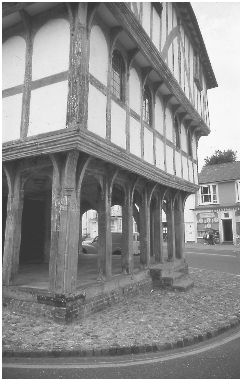
The Guildhall, Thaxted, Essex. A medieval three-storeyed frame in oak, with a double jetty on three sides.
