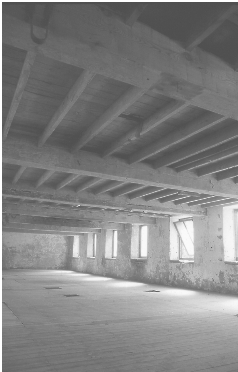
Arkwrights Mill building at Cromford Mill, Derbyshire. Dating from around 1780, this is possibly the world's first factory, with stone walls supporting timber floors of large redwood principals.
