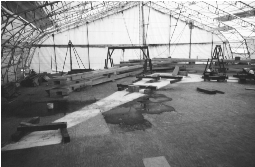
Fig. 18.7.10 The first temporary cover, re-used as the workshop. Two trusses have been fabricated and moved clear of the fabrication outline drawn on the floor
