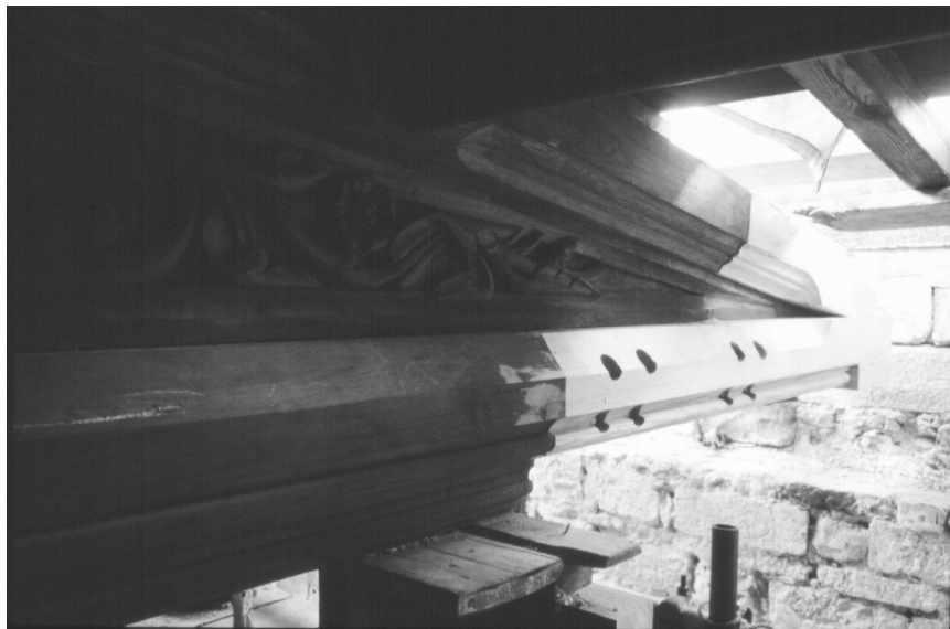
Fig. 12.5 A vertical splayed scarf with bolts and split rings used in Cranbrook Church, Kent. (a) The joint before assembly, showing the bolts and split rings. (b) The assembled joint. (The boltholes are still to be plugged, and the bottom moulding added)
