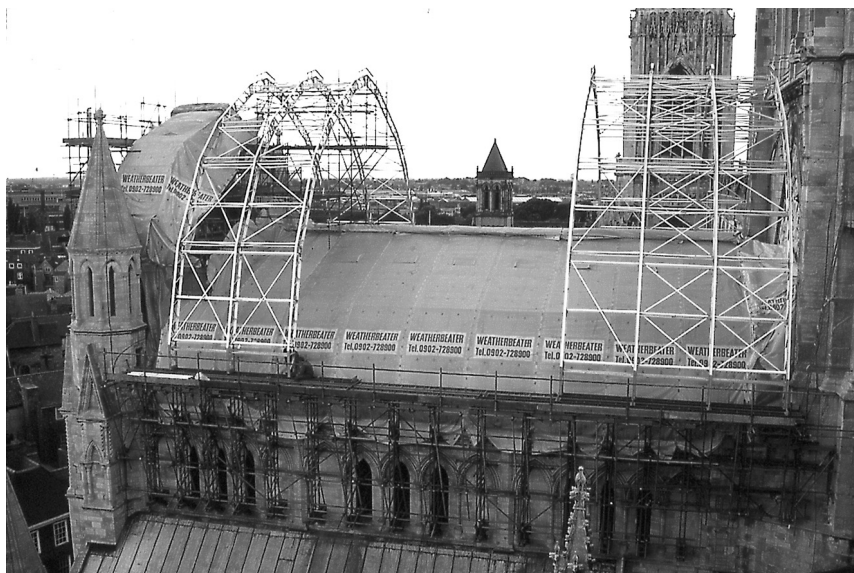
Fig. 18.7.9 The first temporary roof cover, with the second in process of assembly over it
