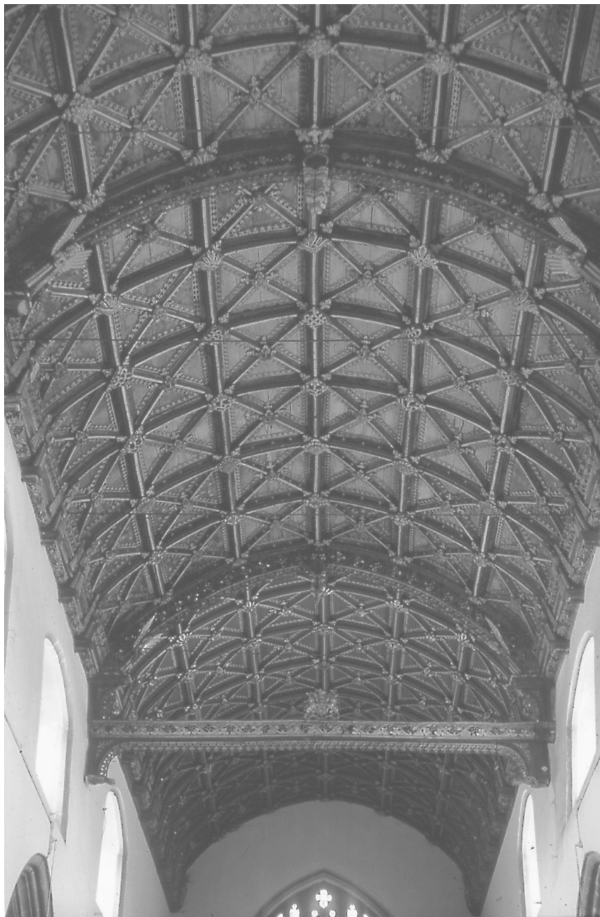
St Andrew's Church, Cullompton, Devon. Seven-cant trusses above, with a barrel vault below.
