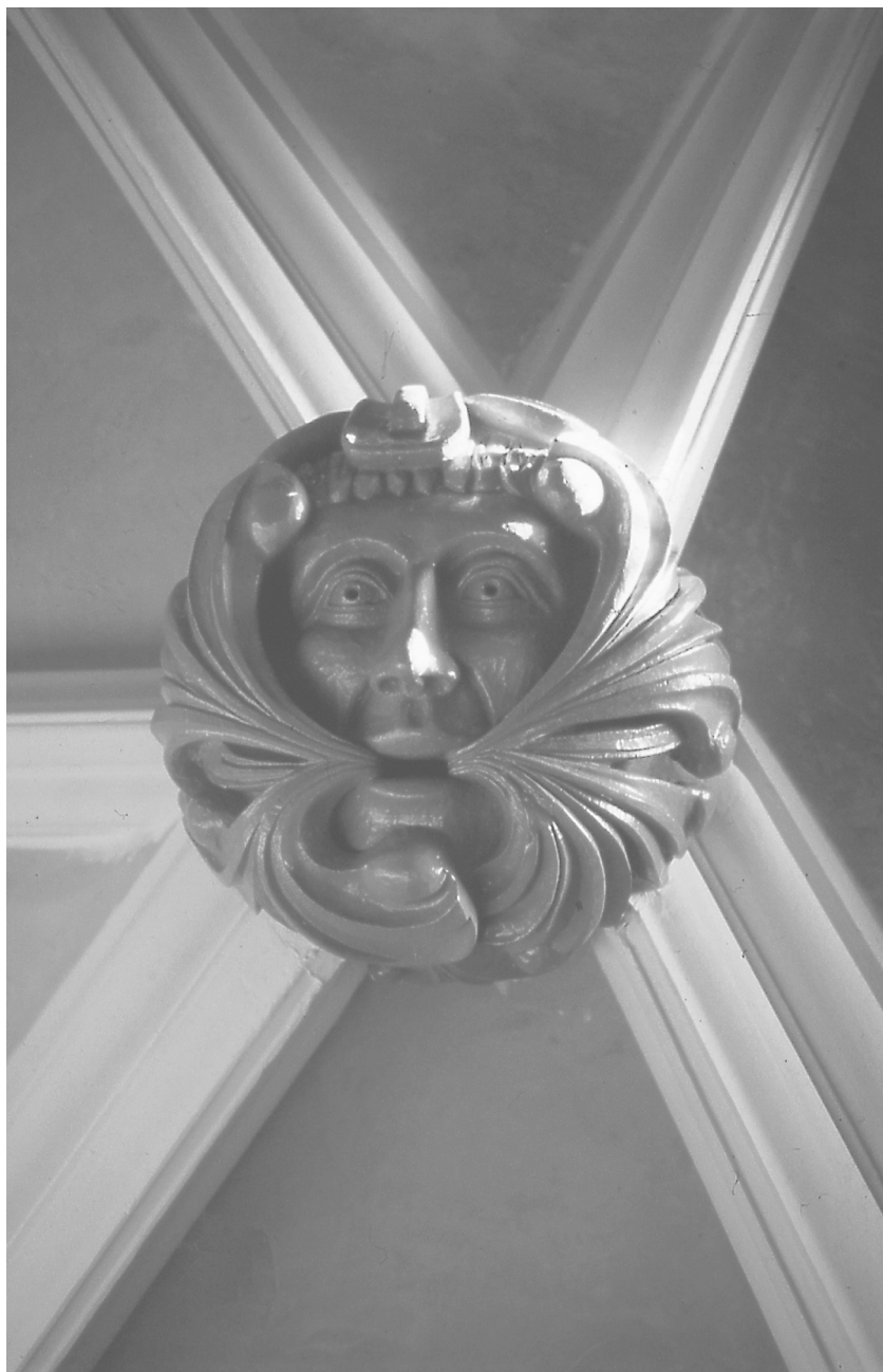
York Minster, South Transept, new roof boss. A representation of the 'green man', carved from a block of laminated oak.
