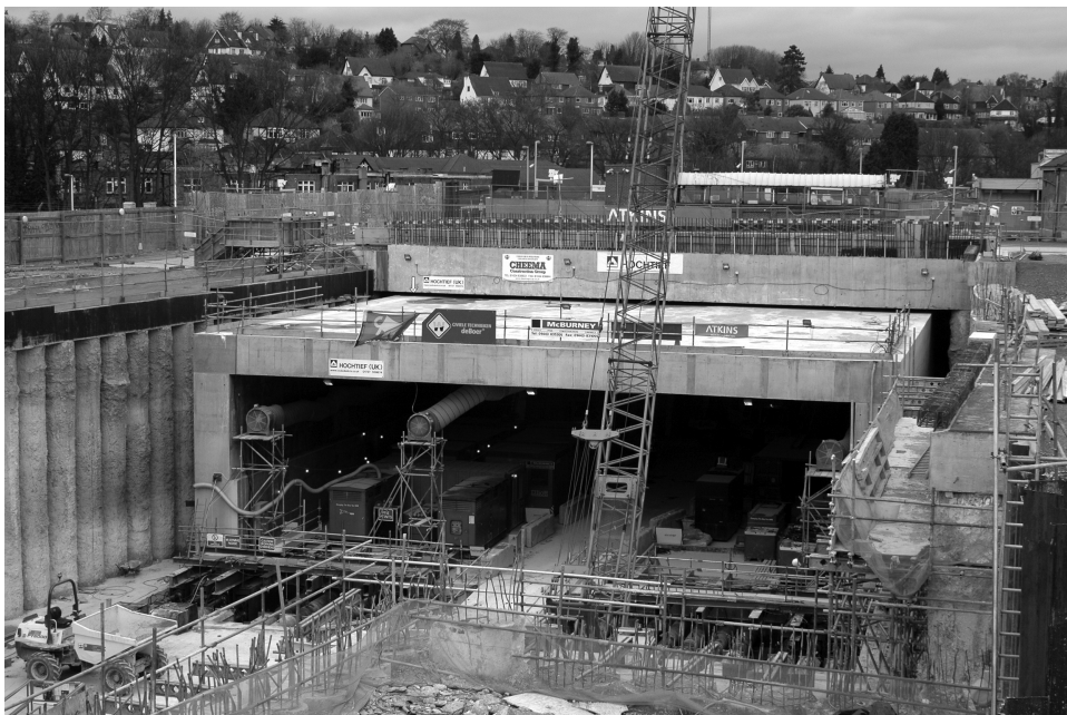
Figure 5.13 Jack box tunnelling beneath a working station.
