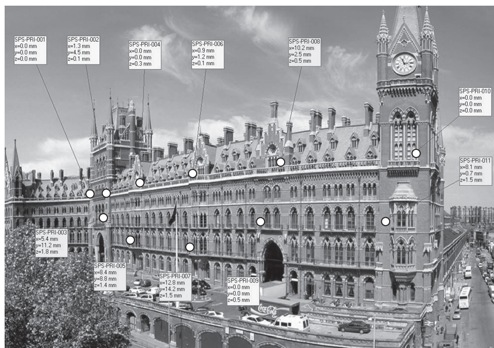
Figure 5.11 The facade of St Pancras Station in London monitored as part of a new London Underground ticket hall excavation below it.
