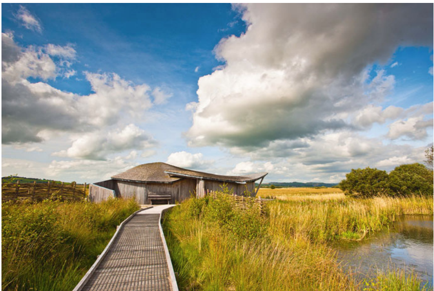
Fig. CS2.7 The new observation shelter
