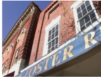
Figure 6.38. Taller second stories are found on the first two buildings. These floors are about 15 feet. The total height for the first two buildings is about 25 feet.
