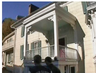
Figure 6.40. A closer view of the residential building reveals that the two levels are partially above street level (approximately 4 feet). The two residential floors are approximately 8 feet each. The total height is approximately 20 feet.
