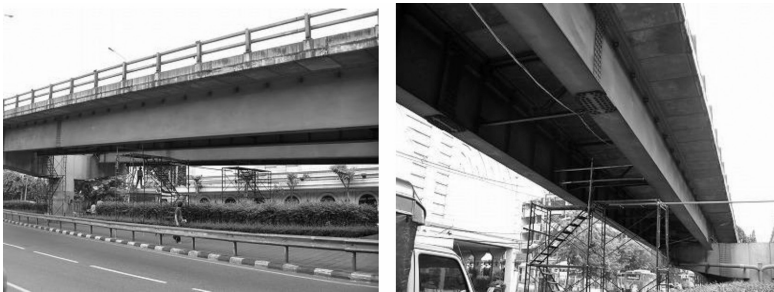
FIGURE 6.19 Monitored bridge: two independent superstructures stay on common piers.
