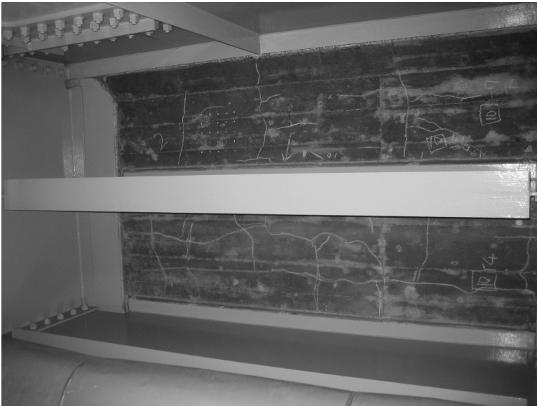
FIGURE 6.12 (See color insert.) Fatigue cracks of a concrete slab (left) and cross beam (right) in Japan.
