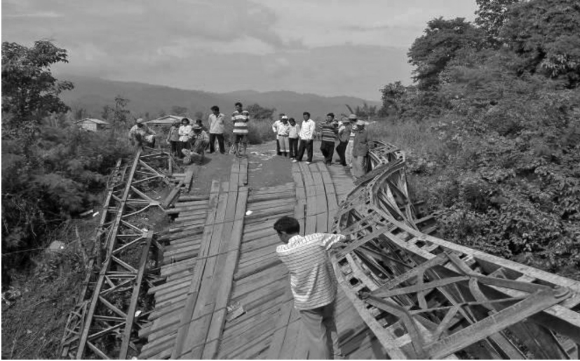
FIGURE 6.11 Bridge collapse in Cambodia (Bailey Bridge).
