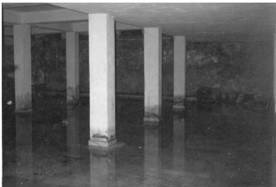
Figure 2. Basement of a house in the old city flooded by rising groundwater levels.
