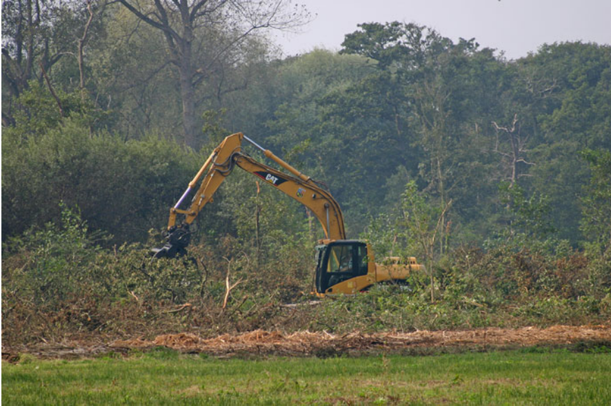
Fig. 9.5 Removing dune scrub and woodland from a former tidal beach plain of the medieval Yser estuary between Nieuwpoort and Oostduinkerke to restore dune slacks in Belgium, picture taken in 2005 (Herrier et al. 2005)
