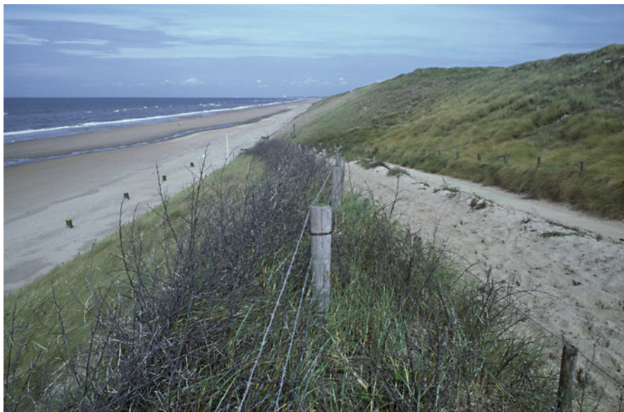
Fig. 6.7 ‘Fixed’ steep-faced coastal dune defences in the Netherlands, 1987
