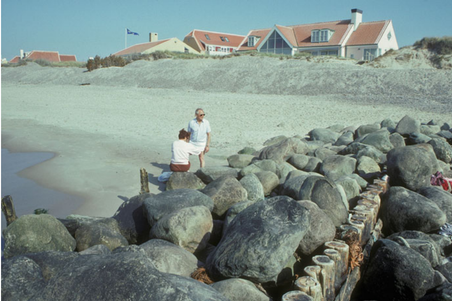
Fig. 6.6 Hard defences ‘protecting’ sea front houses built on sand, Jutland, Denmark 1992. It appears as though sand from the beach has been used to augment the dune ridge seaward of the houses
