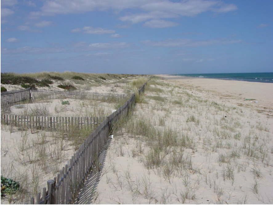
Fig. 9.1 Grid chestnut paling fencing on a coast apparently with a positive sediment budget, Algarve near Faro 2005
