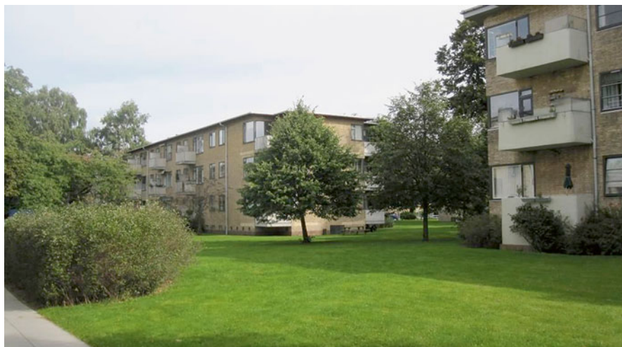
Fig. 5 Photo taken 2009 of some of the houses in the Blidah-park
