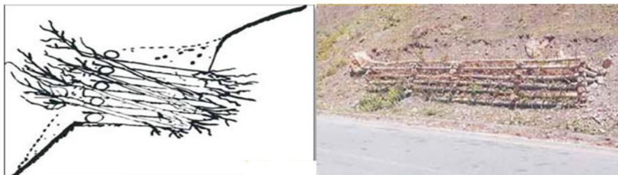
Fig. 8.4 Vegetated timber crib wall
