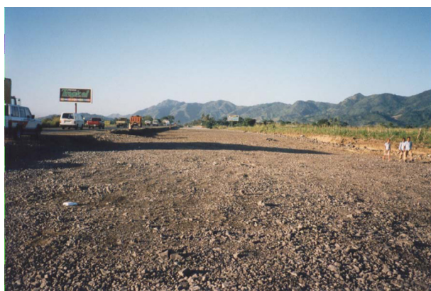
Fig. 8.6 Blended crushed river gravel and Falcondo aggregate (nickel slag) granular base use for Autopista Duarte widening near Bonao.
