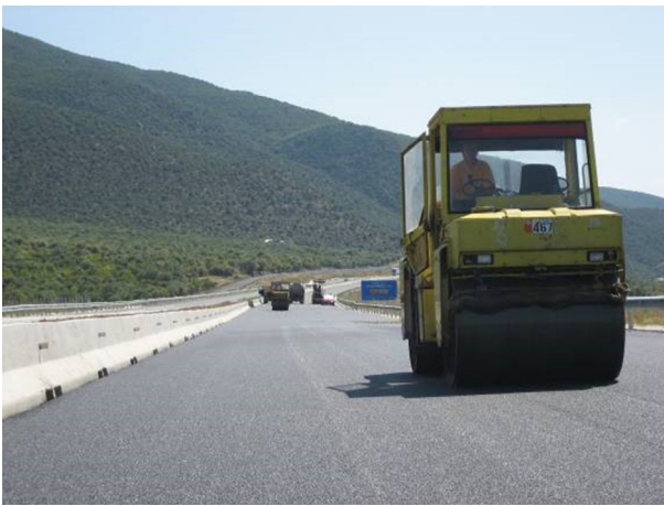
Fig. 14.3 Mix compaction.
