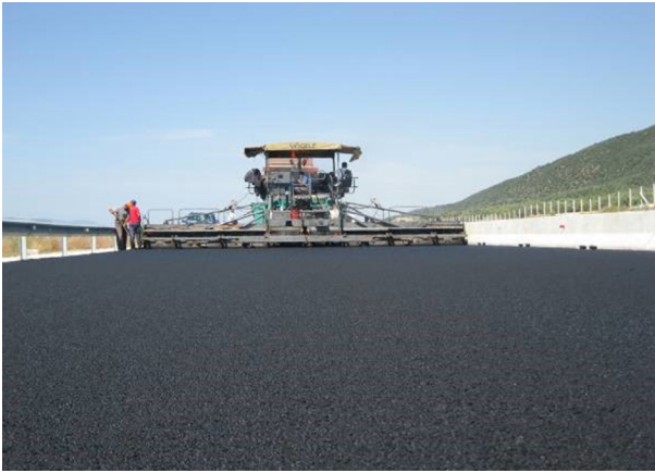
Fig.14.2 Asphalt paving.
