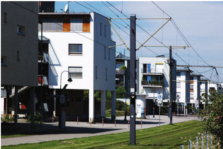
Figure 5.10. View of commercial building ends in Vauban. (Photograph by Transurban: Thomas Schroepfer and Christian Werthman, with Limin Hee.)
