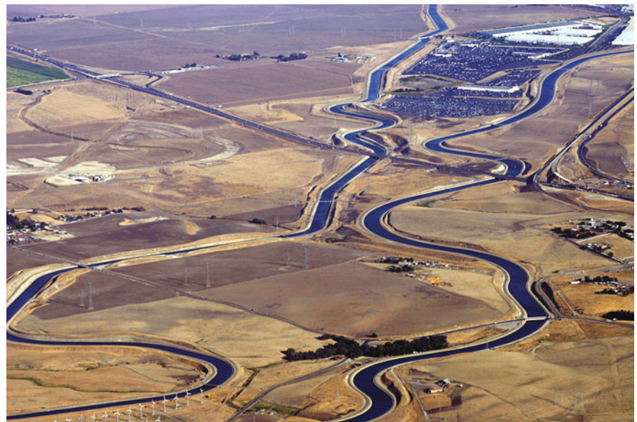
Figure 7.9. California's water infrastructure. (Photograph by Ian Kluff.)
