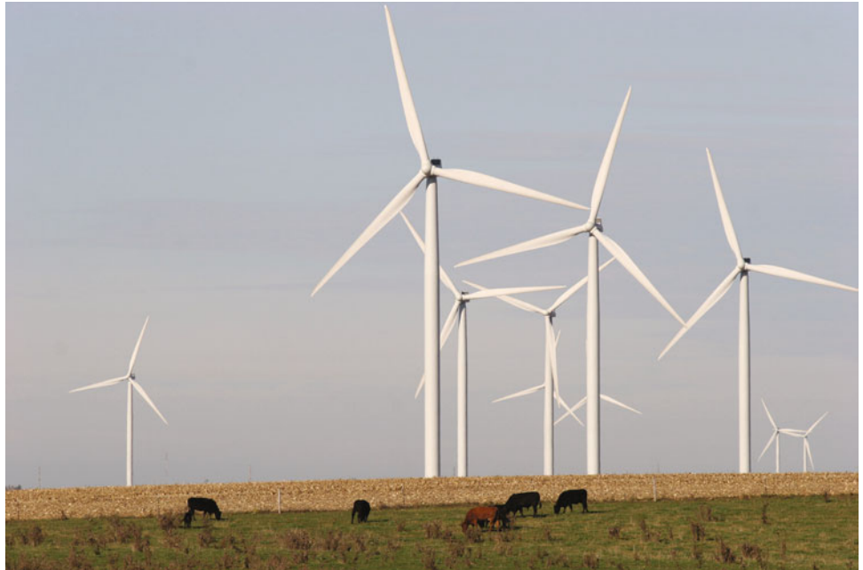
Figure 7.2. View of wind farm. (Photograph by Argonne National Laboratory.)
