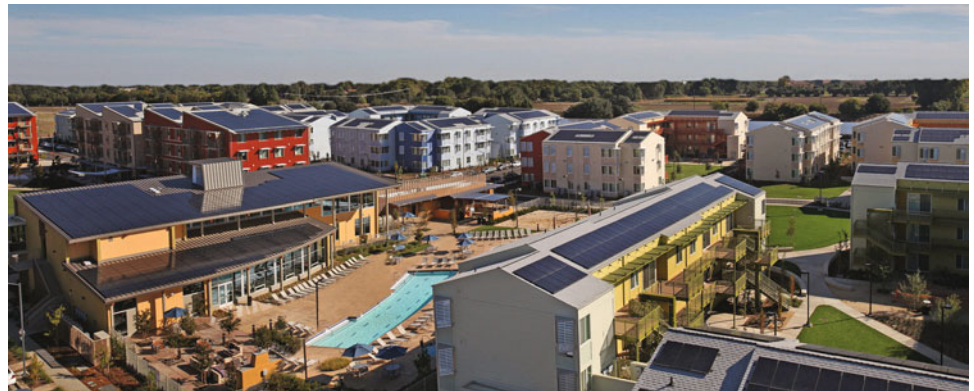
Figure 7.26. View of photovoltaic arrays on roofs in West Village. (Photograph by West Village Community Partnership.)
