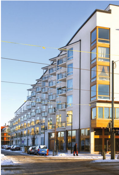
Figure 3.14. View of balconies facing the lake in Hammarby Sjöstad. (Photograph by Lennart Johansson.)
