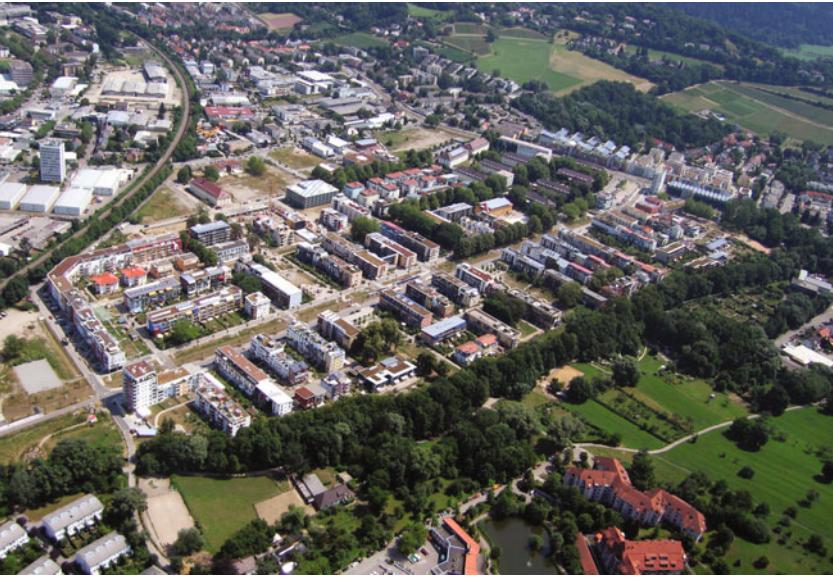
Figure 5.1. Aerial view of Vauban, Freiburg, Germany. (Photograph by Transurban: Thomas Schroepfer and Christian Werthman, with Limin Hee. )
