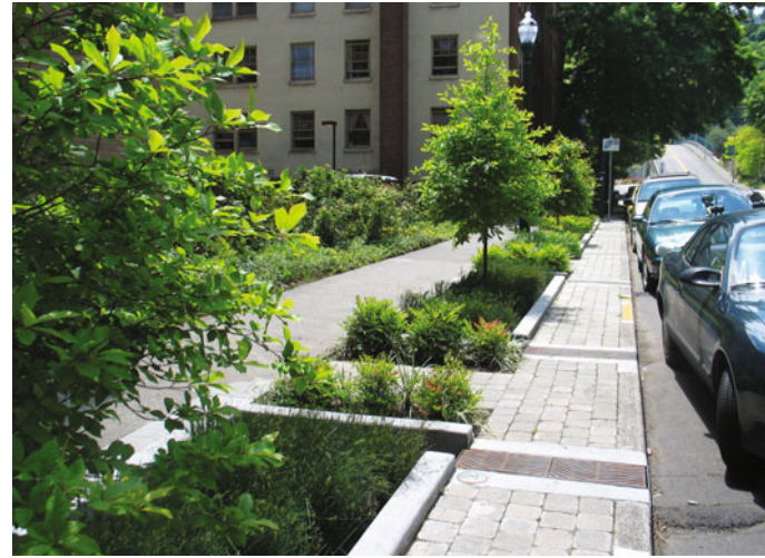
Figure 7.10. View of storm-water planters, SW 12th and Montgomery Streets, Portland, Oregon. (Photograph by Environmental Services, City of Portland.)
