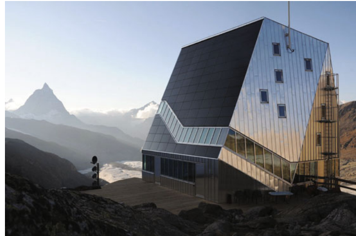
Figure 7.7. View of photovoltaics on a facade, Monte Rosa, Switzerland. ( Photograph by Sunpower Inc. )
