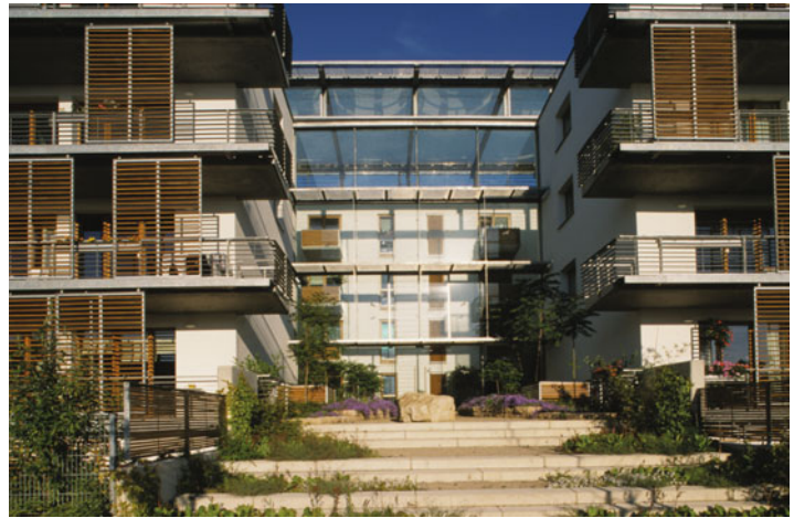
Figure 4.24. View of microclimate zone east-side entrance in Kronsberg. (Photograph by Karl Johaentges.)
