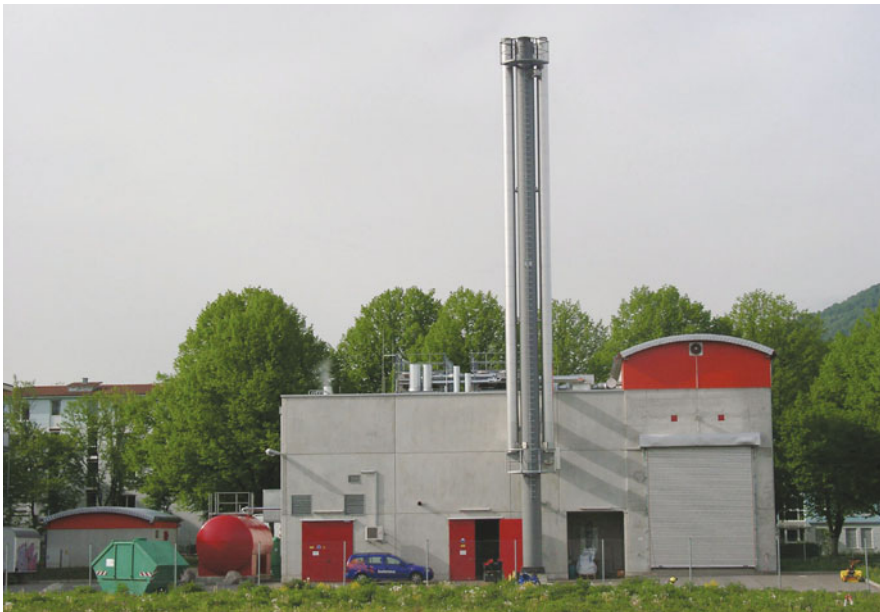
Figure 5.22. Cogeneration Plant 1 in Vauban. (Photograph by Carsten Sperling.)
