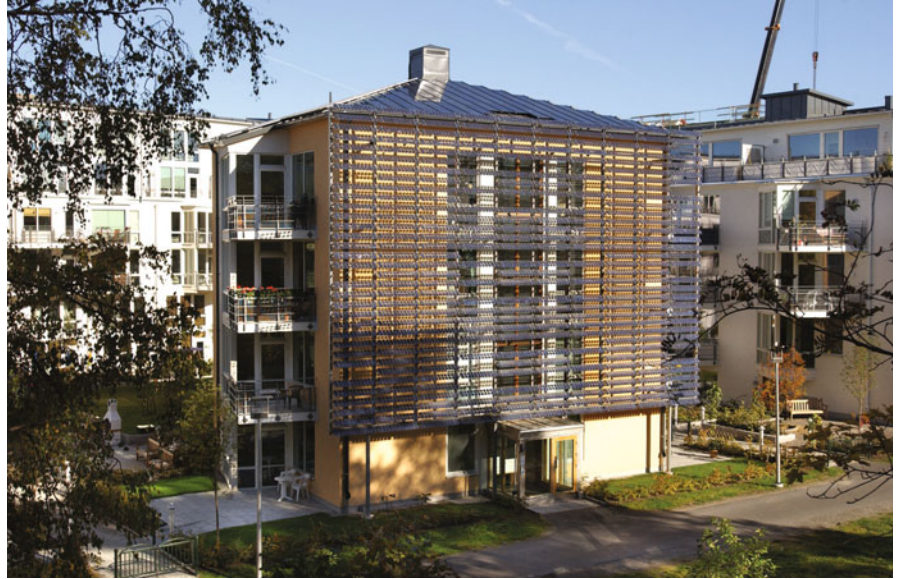
Figure 3.20. View of photovoltaic facade screen in Hammarby Sjöstad. (Photograph by Lennart Johansson.)
