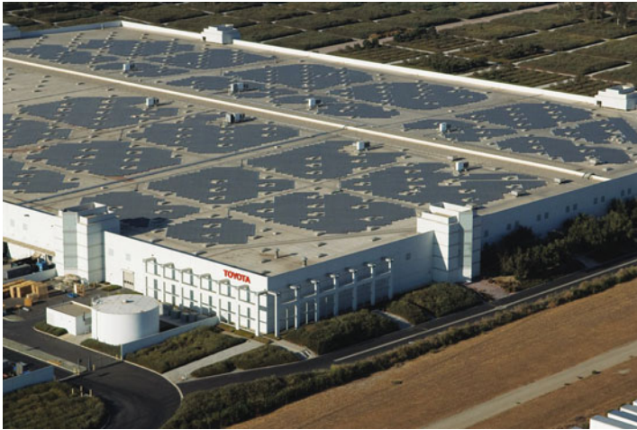
Figure 7.6. View of photovoltaics on a roof, Ontario, Canada. ( Photograph by Sunpower Inc. )
