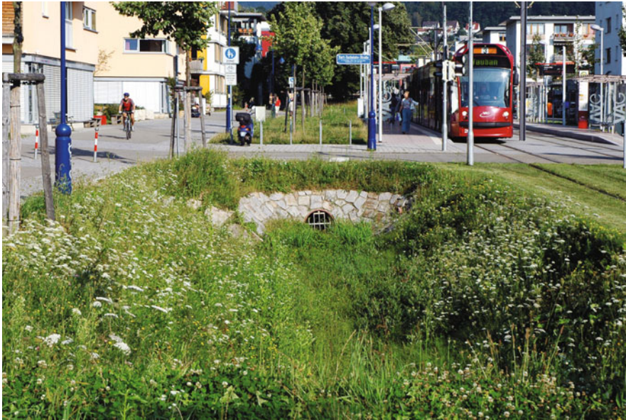
Figure 5.26. View of central storm-water swale in Vauban. (Photograph by Transurban: Thomas Schroeppfer and Christian Werthmann, with Limin Hee.)
