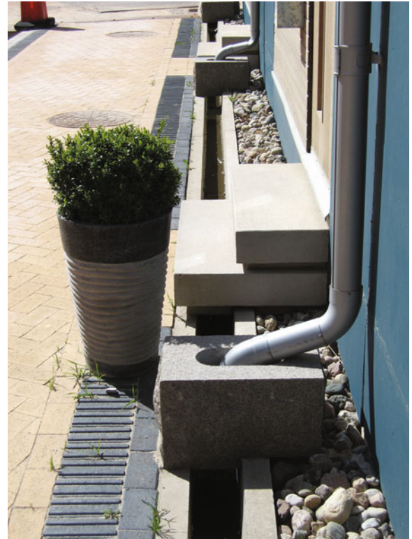
Figure 2.15. Storm-water downspout in Boo1. (Photograph by Bengt Persson.)
