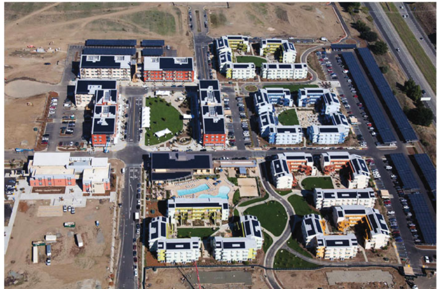
Figure 7.29. Aerial view of West Village. (Photograph by West Village Community Partnership.)
