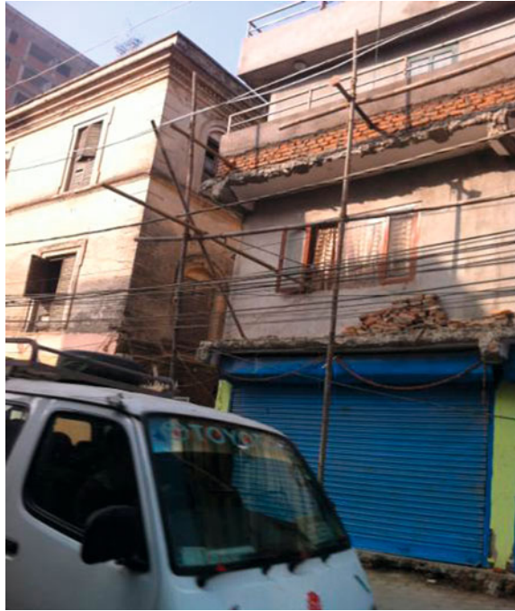
Fig. 2.6 Scaffolding in Kathmandu, Nepal (Photograph by author, 2013)
