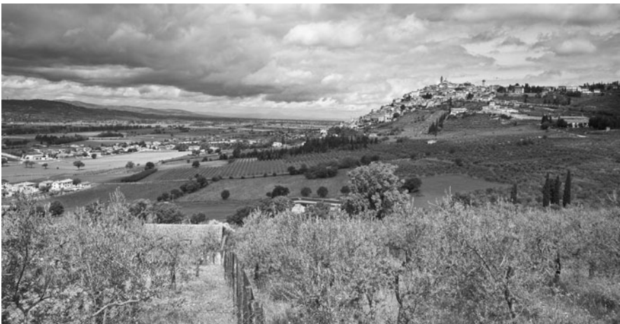
Fig. 4.18 Trevi, Umbria. The relationship between the historic city and the infrastructure of the plain situated below it
