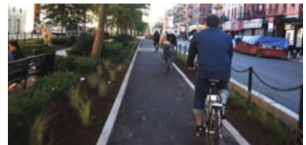
NEW YORK, NY A cycle track takes advantage of the central median and insulates cyclists from double parking.
