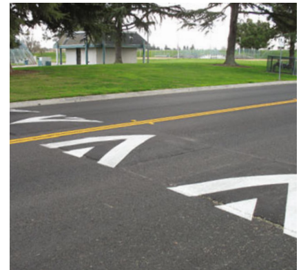
Speed cushions allow emergency vehicles to pass their wheels on either side of the raised area.
