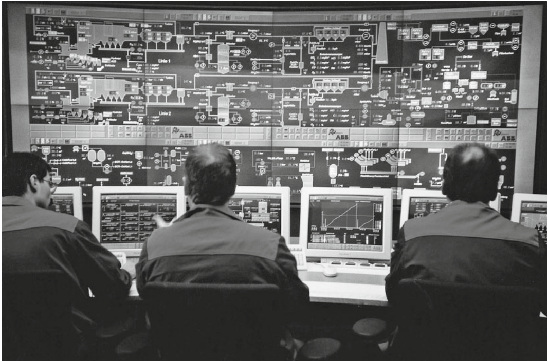
Control room of a moving grate incinerator for municipal solid waste, Germany
