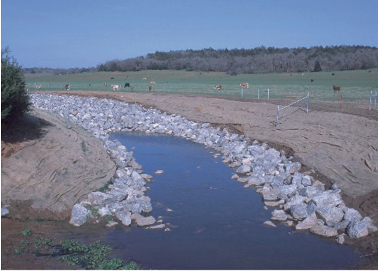
Plate 44 Grade stabilization structures are established along drainageways to prevent gully erosion (Courtesy USDA-NRCS)
