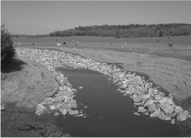
Fig. 11.2 Grade stabilization structures are established along drainageways to prevent gully erosion (Courtesy USDA-NRCS)
