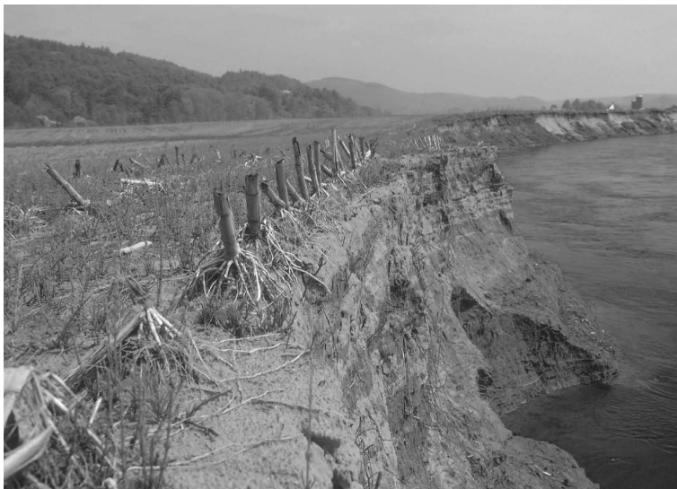
Fig. 2.3 Corn field severely affected by streambank erosion (Courtesy USDA-NRCS). Saturated soils along streambanks slump readily under concentrated runoff, which causes scouring and undercutting of streambanks and expansion of water courses
