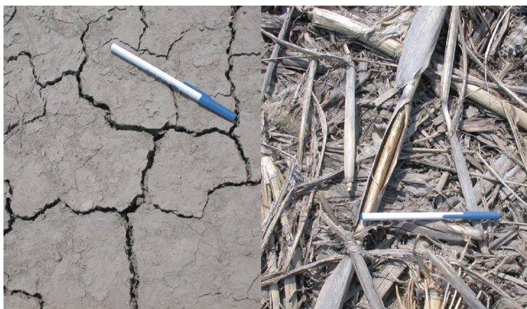
Plate 16 Crop residues protect soil from cracking, crusting, and surface sealing (Photo by H. Blanco)
