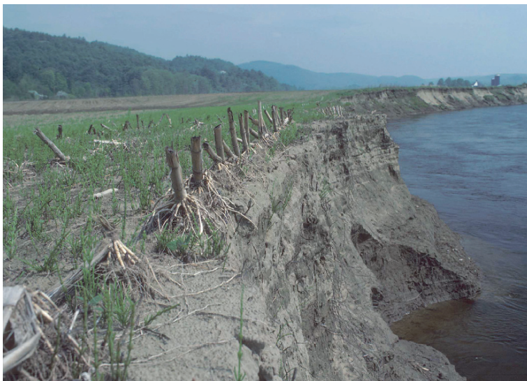
Plate 8 Corn field severely affected by streambank erosion (Courtesy USDA-NRCS). Saturated soils along streambanks slump readily under concentrated runoff, which causes scouring and undercutting of streambanks and expansion of water courses
