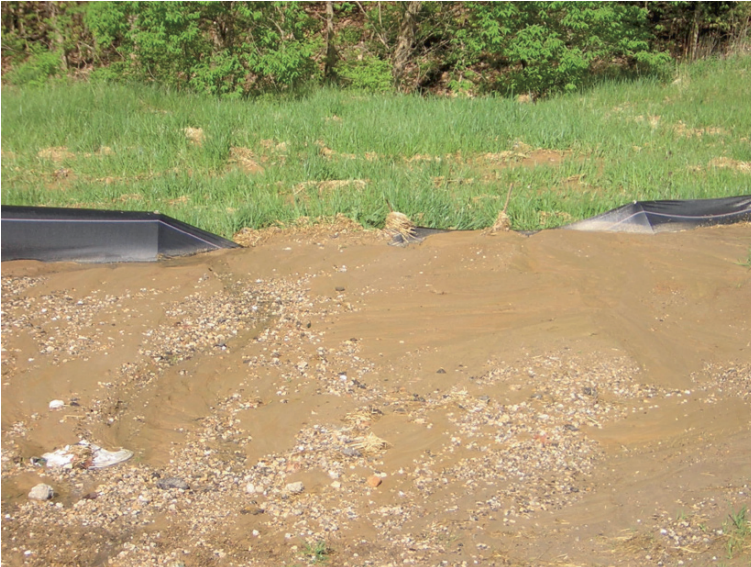
Plate 43 Sediment accumulation above silt fences can overtop them under concentrated flow erosion (Courtesy C.J. Gantzer Univ. of Missouri)
