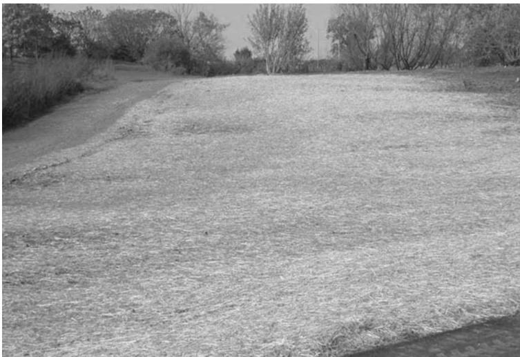
Fig. 12.11 Disturbed area seeded to grass under mulch cover (Courtesy Ryan Bartels)
