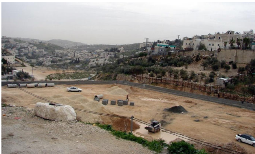
Construction of the new football grounds in Jabel Mukaber
