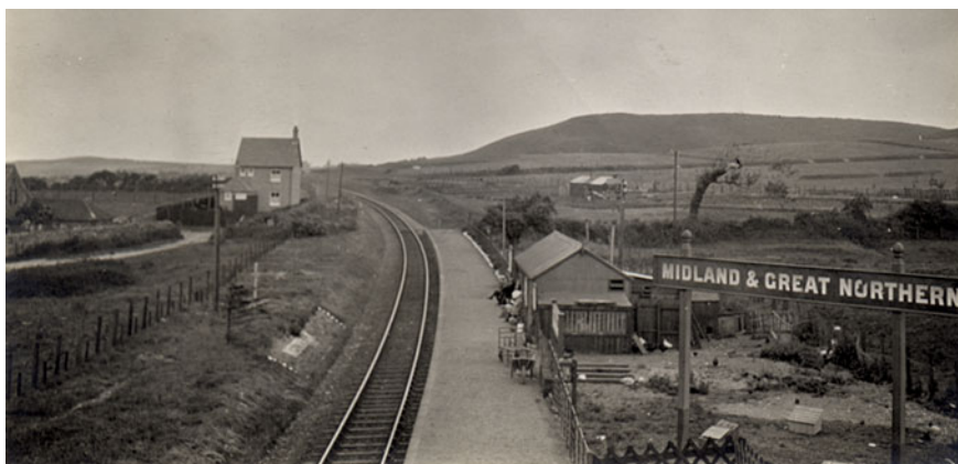
Fig. 3.29 P680291 (1907) Harmer's geological excursion to Norfolk. Looking west along the former Midland & Great Northern Railway line between Mundesley and Weybourne with hummocky drift features in the background near Sheringham. Harmer noted that such knoll-like landforms are also common in other glaciated areas of northern Europe (Harmer 1910a, b). (CP13/050 Reproduced by permission of the British Geological Survey © NERC. All rights reserved)
