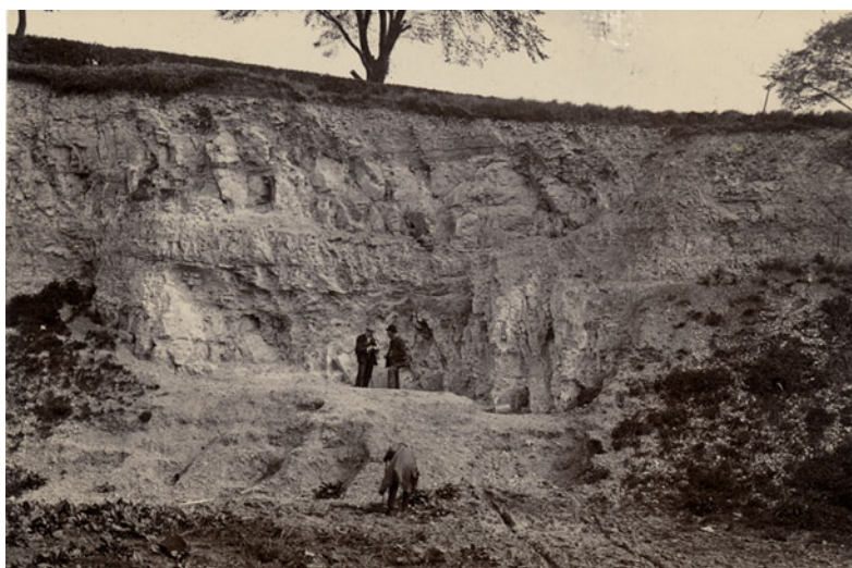
Fig. 3.19 P680272 (1907) A chalk quarry exposing the Cretaceous bedrock that forms the solid geology of Norfolk; dipping from west to east this formation comprises the top of cliffs at Hunstanton, the base of the cliffs at Weybourne and lies at about 150 m (500 ft.) below sea level at Great Yarmouth. (CP13/050 Reproduced by permission of the British Geological Survey © NERC. All rights reserved)
