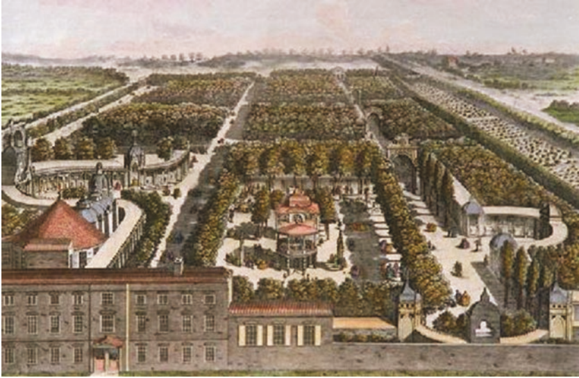
Fig. 2 ‘A General Prospect of Vaux Hall Gardens, Shewing at one View the disposition of the whole Gardens’. Engraving by Johann Sebastian Müller after Samuel Wale, 1751. Courtesy of David Coke collection
