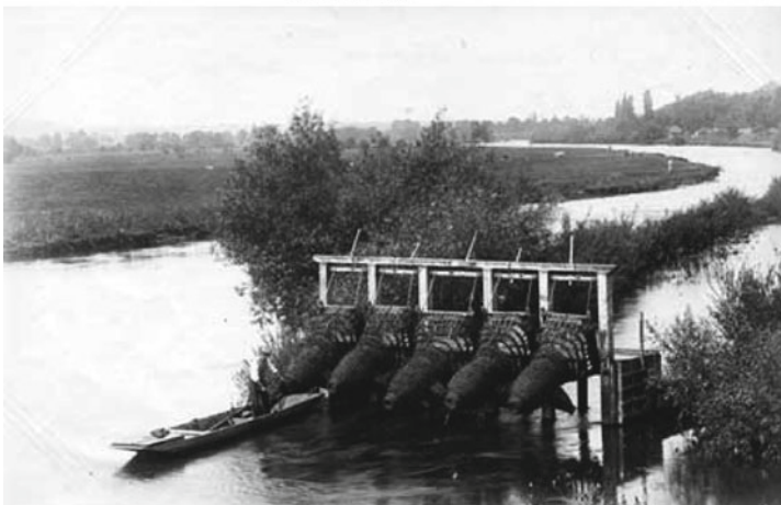
Fig. 1.6 An illustration ( top left ) of eel bucks, large wicker baskets that can be lowered into a flowing river to catch silver eels. Examples of these are documented in nineteenth century photographs at Harleyford
