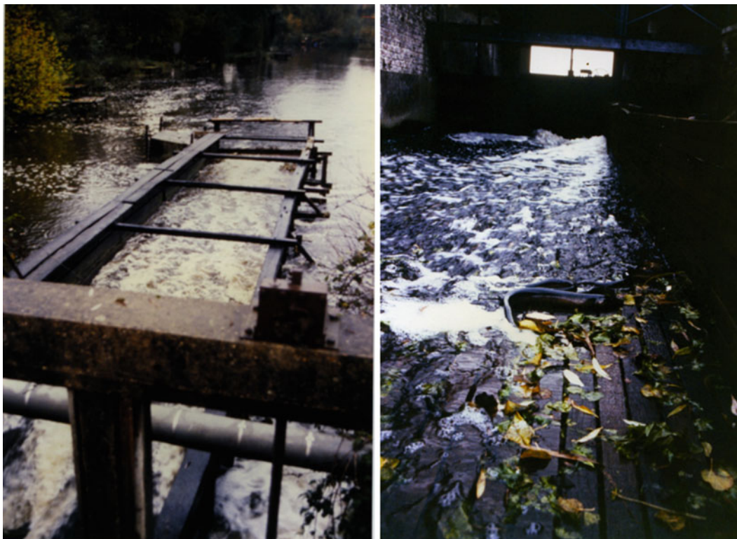
Fig. 5.14 Anguillères (eel gears) used in the Bay of Somme, northern France. Photographs courtesy Antoine Legault, Fish-Pass, reproduced with permission
