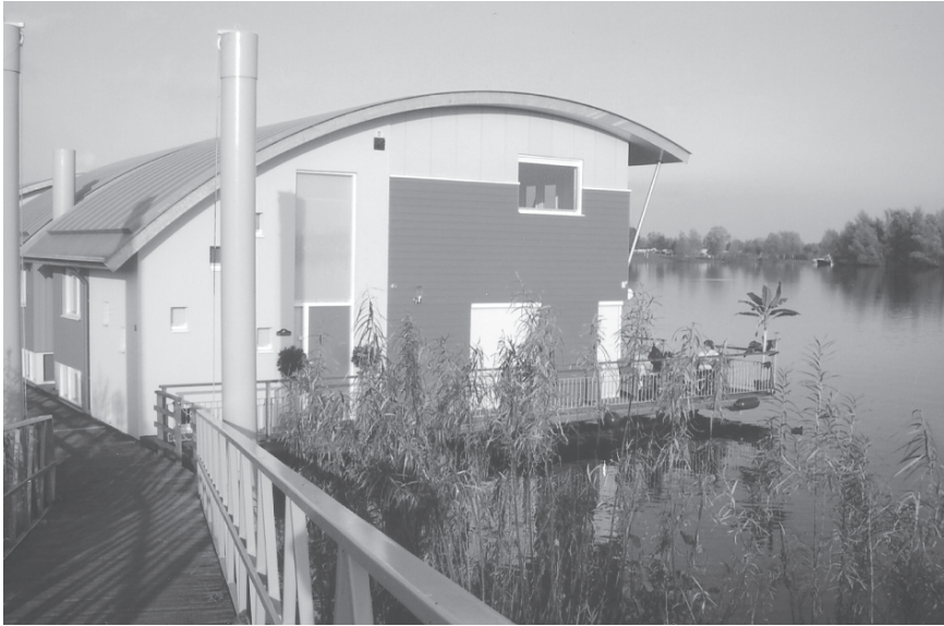
Fig. 21.6 Housing in the future: solid real estate will become floating real estate. Floating houses in Maasbommel on the river Maas, November 2005 (Photograph P.H. Nienhuis)
