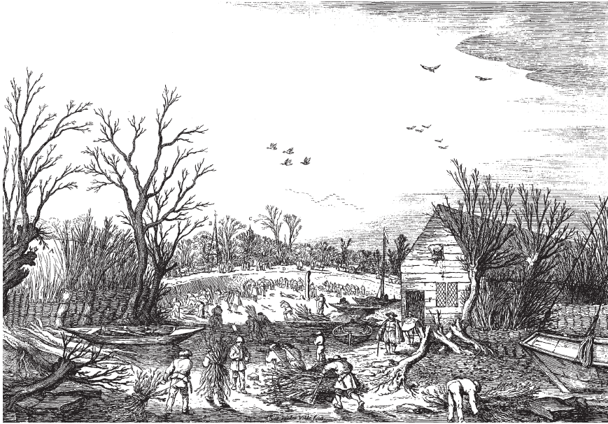
Fig. 9.10 Repair of the breached dyke of the river Lek after the ice jam of January 10, 1624. Dyke workers are engaged in closing off the breach by means of a 'vingerling'. To the left a part of the old dike with wattle-work is reinforced with faggots. In the centre a new curved stretch of dyke is built ('vingerling') in which numerous fascines are used; on top of the new dyke charts pulled by horses (Drawing by the contemporary artist Esyas van den Velde)
