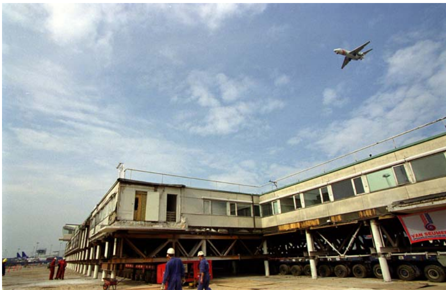
The recently restored airport terminal in Copenhagen houses the administrative offices for all of the airport’s employees. Quality is expressed in many ways – one of which is the reestablishment of the original entrance with columns and a canopy. The airport terminal was carefully moved to a new location (Photograph: Copenhagen Airport Press Photography)
