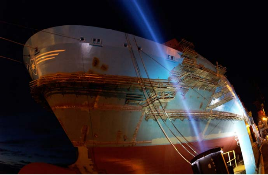
The magnificent Maersk container ship – one of the largest in the world – also symbolized growth. The fact that it was still under construction, combined with the dramatic lighting, contributed to this message (Photograph: 3rdDimension©)
