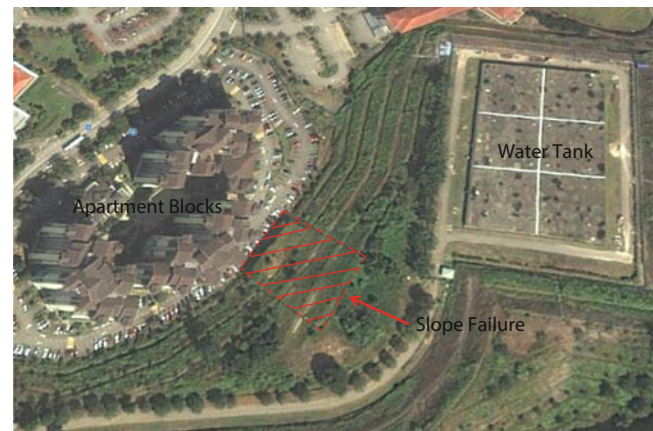
Fig. 1 Location of slope failure in Precinct 9, Putrajaya
