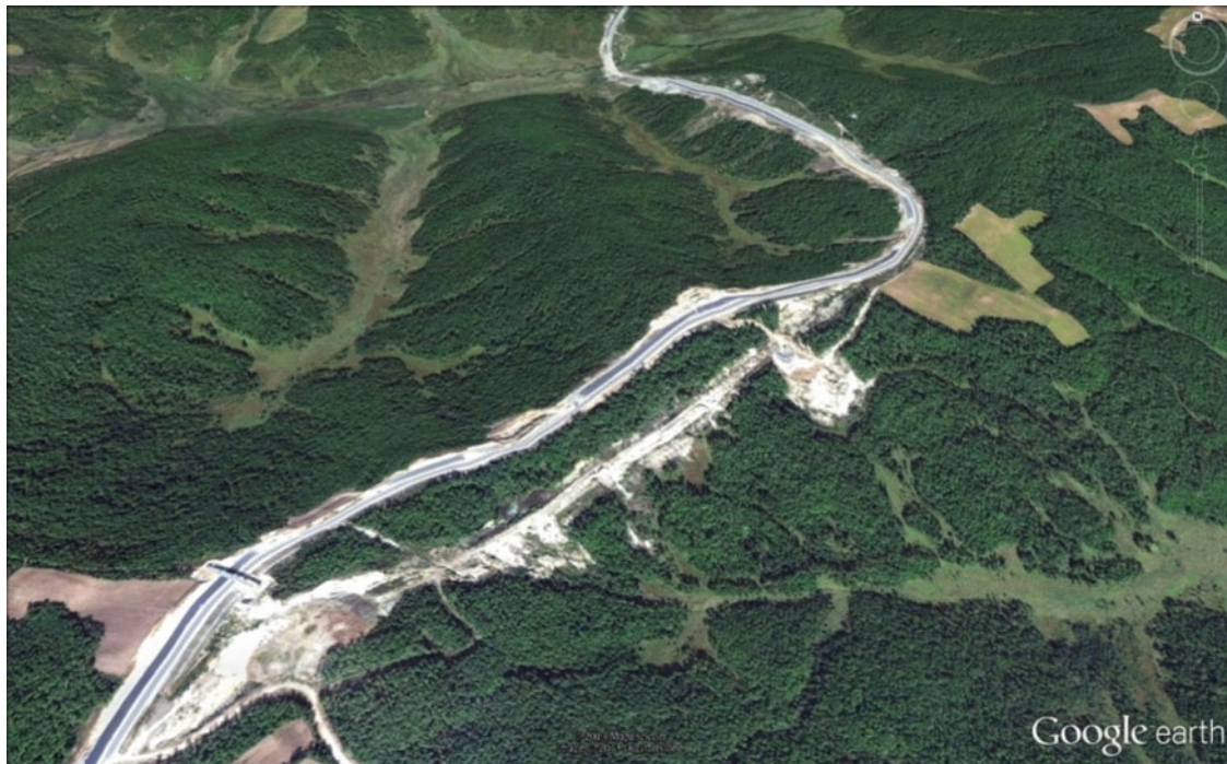
Fig. 1 Aerial view of the Bei'an to Heihe Expressway expansion project
