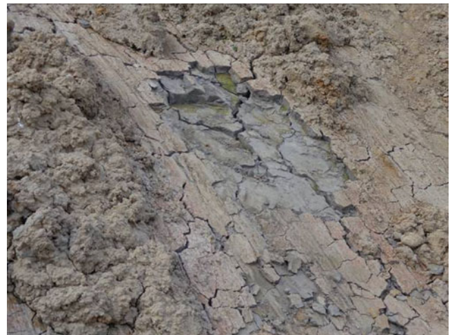
Fig. 9 Exposed slickensides observed throughout the landslide area
