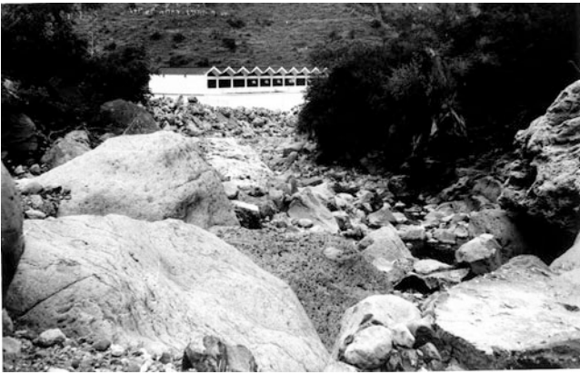
Fig. 7 View on the powerhouse from the Hako Creek valley after the disaster
