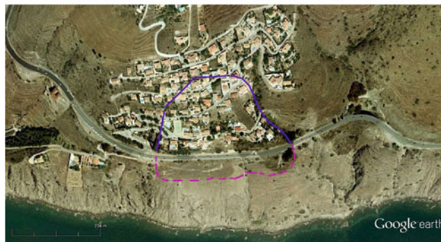
Fig. 9 Above : An empty exhausted block slide at the Western slope of Cerro Gordo; Middle : An urbanization built up on the previously existing Calaiza landslide in the Eastern slope of Cerro Gordo, causing damaging consequences. Below : slide on Alfamar urbanization. See Fig. 4 for setting of these examples
