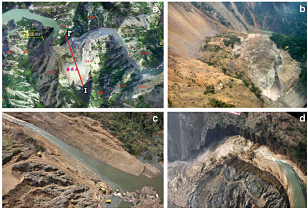
Fig. 3 Tangjiashan landslide dam. (a) Aerial view; (b) view of the dam body; (c) view of the dam after construction of spillway (June 8, 2008); (d) view of the dam body with sudden breaching on June 10, 2008
