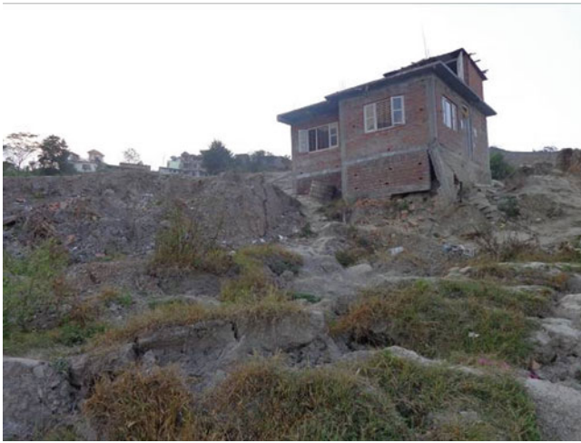
Fig. 6 Damage to the house that was swept away by the landslide
