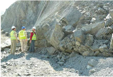
Fig. 2 Example of debris accumulated at the bottom of a fixed drapery system
