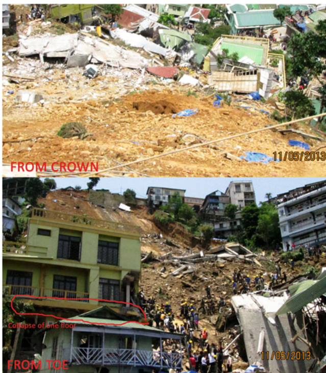
Fig. 8 Effects of rockslide
