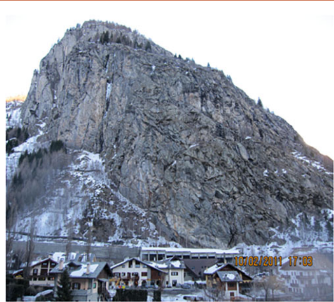
Fig. 1 South-western slope of Mont La Saxe susceptible to rockfall. At the bottom of the slope, the endangered village, the main national road, and the old rock shed are visible
