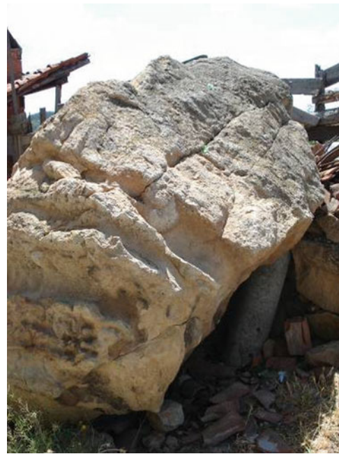
Fig. 2 A large fallen block stopped by a street lamp and garden wall in the southwestern foothill of the castle
