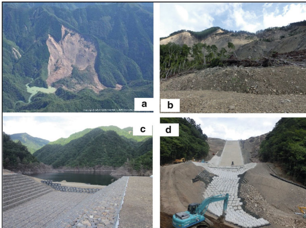
Fig. 9 Kuridaira landslide dam. (a) Aerial view (Photo courtesy of Aero Asahi) of the site few hours after the landslide was formed. (b) Front view of the main scarp and main sliding body. (c) Stabilized
