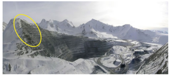
Fig. 1 General view of the pit as of 2008: the yellow ellipse shows the collapse area in the upper north-eastern part of the pit area in 2002 and 2006
