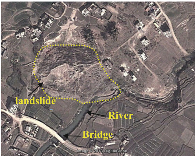
Fig. 2 Google Earth photograph of the landslide
