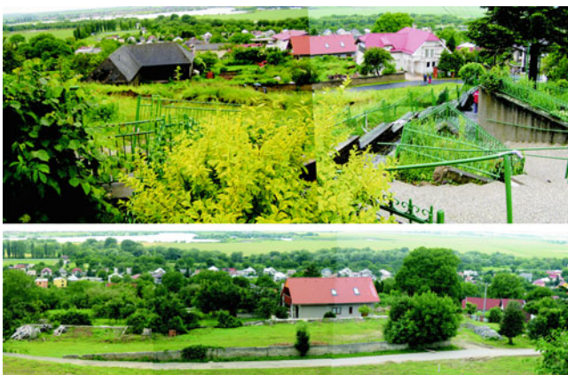
Fig. 6 Panoramic view of the central part of the Nižná Myšľa Village destroyed by the catastrophic landslide on 4th June 2010 and the same area after remedial measures (Photo: L'. Petro)
