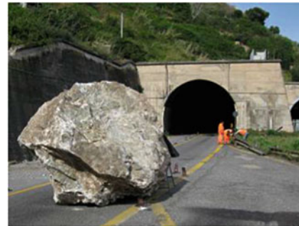
Fig. 5 Large block fell on the Highway A3 at km 425 (2010—Italy)
