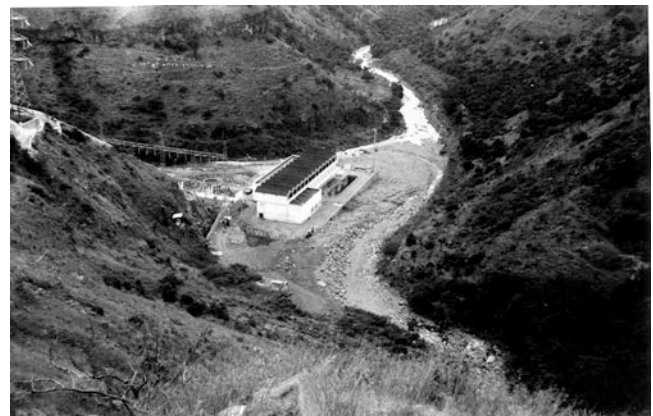
Fig. 6 1991 Debris flow deposits at the Malka Wakana powerhouse
