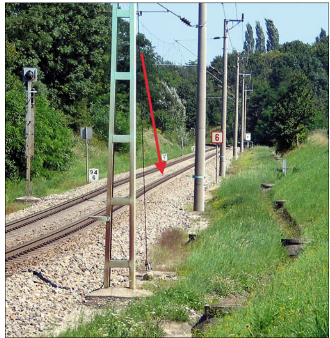
Fig. 2 Current deformation (red arrow) of the railroad tracks of the “Raaberbahn” caused by the activity of the complex landslide L1. Strong deformation of the drainage trench is also visible
