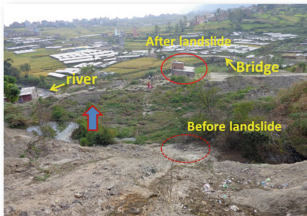
Fig. 3 Overall view of the landslide area
