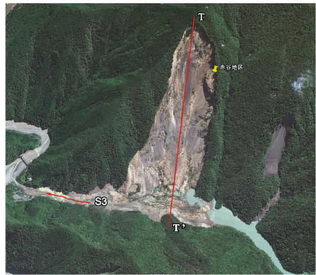
Fig. 5 Akatani landslide dam (Google Earth image) and geophysical survey line (S3)
