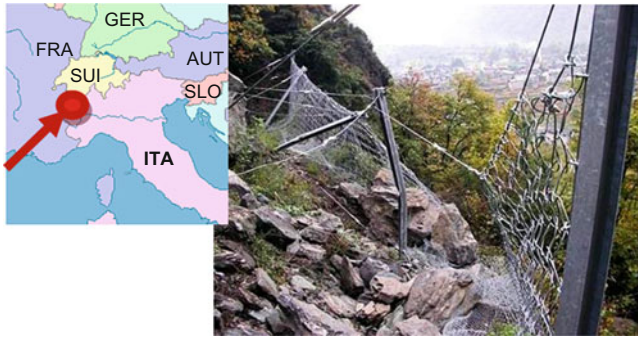
Fig. 10 3,000 kJ barrier impacted by an energy higher than the nominal one. Location: Arnad (Aosta, Italy—2008)
