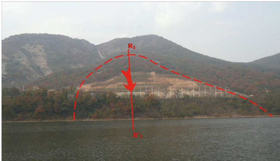
Fig. 1 General view of Daxishan reservoir landslide
