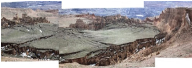
Fig. 7 Graben-shaped separation wall of landslide Old substation
