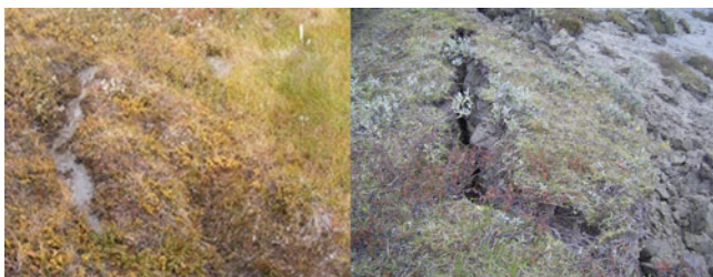
Fig. 3 Crack filled with suspension pressed out due to high pore pressure ( left pane ) and edge crack ( right pane ), Yamal Peninsula
