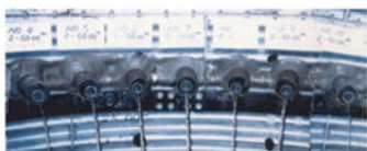
Water catchment boring
