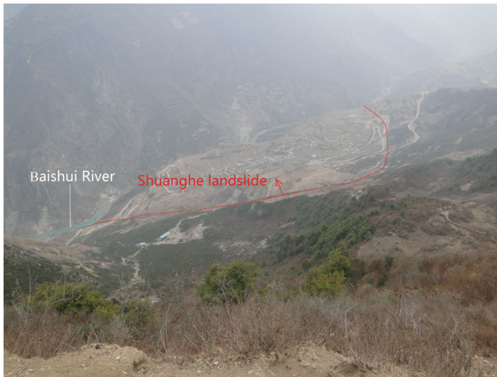
Fig. 5 The whole topography of Shuanghe landslide
