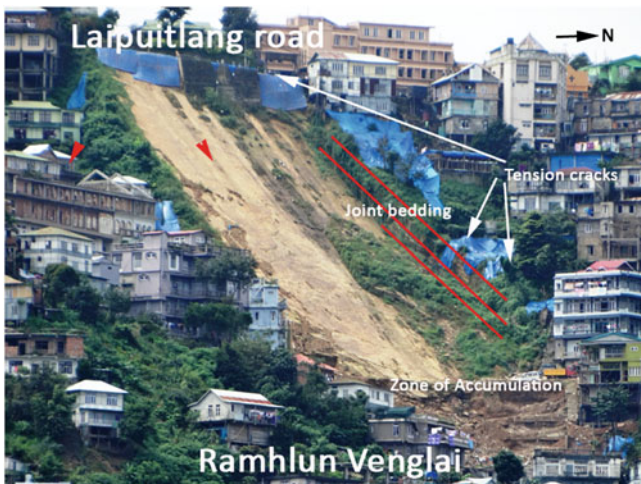
Fig. 4 Photograph showing joint bedding, tension cracks and zone of accumulation
