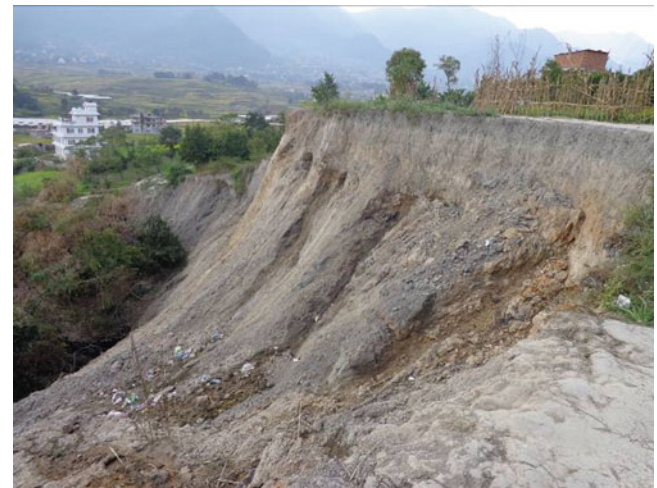
Fig. 5 A view of the side scarp of the landslide
