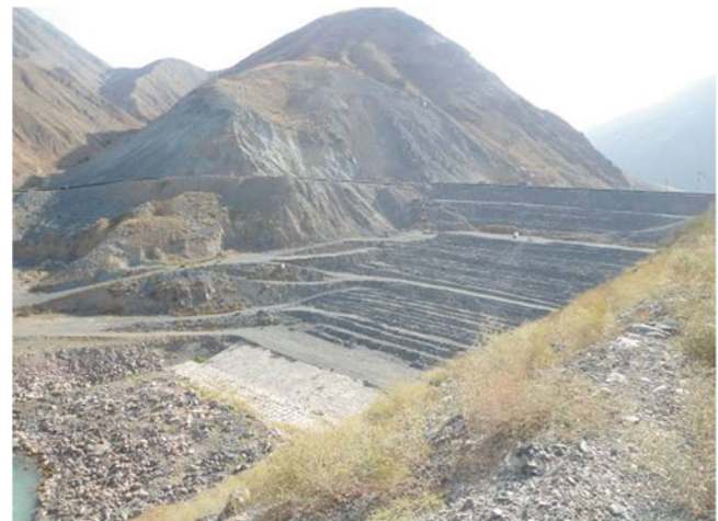
Fig. 2 General view (to the east) of KHPP-2 dam, situated on the Naryn River
