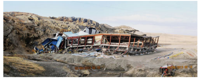
Fig. 3 The view to the front part of the sliding mass (June, 2013), showing the destruction of the administration building and mine infrastructure damage
