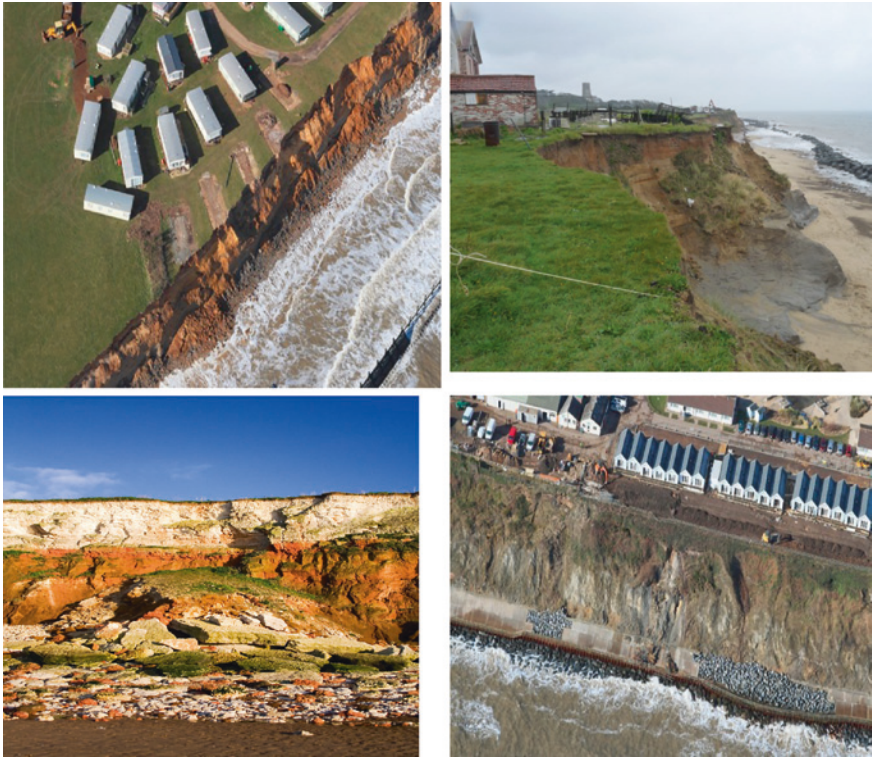
Fig. 2.3 Coastal erosion in east Anglia UK
